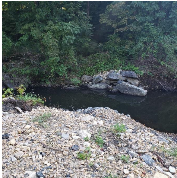
Figure 1: Remnants of Bridge No. 05971 Masonry Abutments
