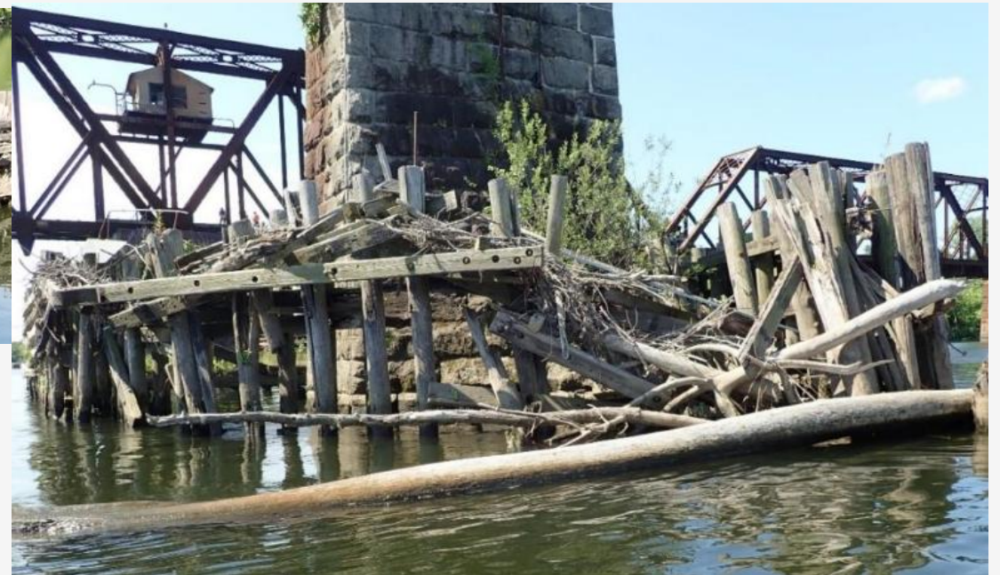
Rehabilitation of Bridge No. 00639R // State Project No. 0082-0317
