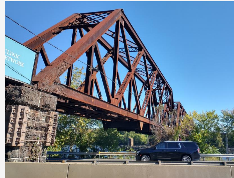
Rehabilitation of Bridge No. 00639R // State Project No. 0082-0317
