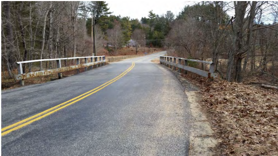
Image 4: Roadway level of Bridge #04730 looking east along Gurleyville Road.
