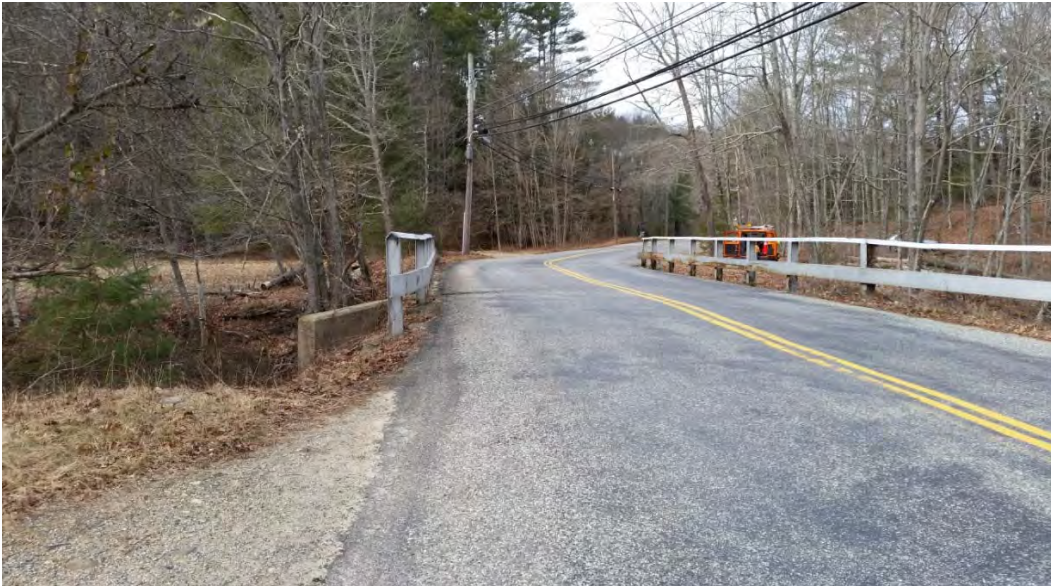
Image 5: Roadway level of Bridge #04730 looking west along Gurleyville Road. Note the existing Nipmuck Trail parking area northwest of the bridge (to be replaced) and the existing gravel parking area southeast of the bridge (to be replaced).
