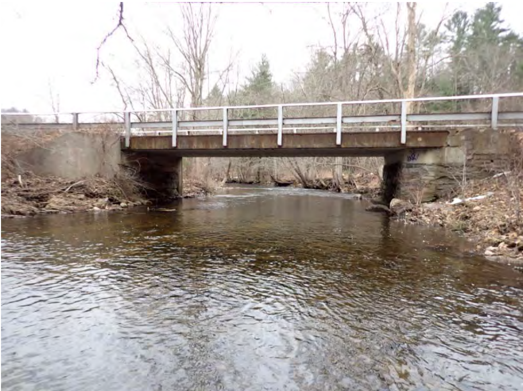
Image 3: North (upstream) face of Bridge #04730 looking south from the Fenton River.
