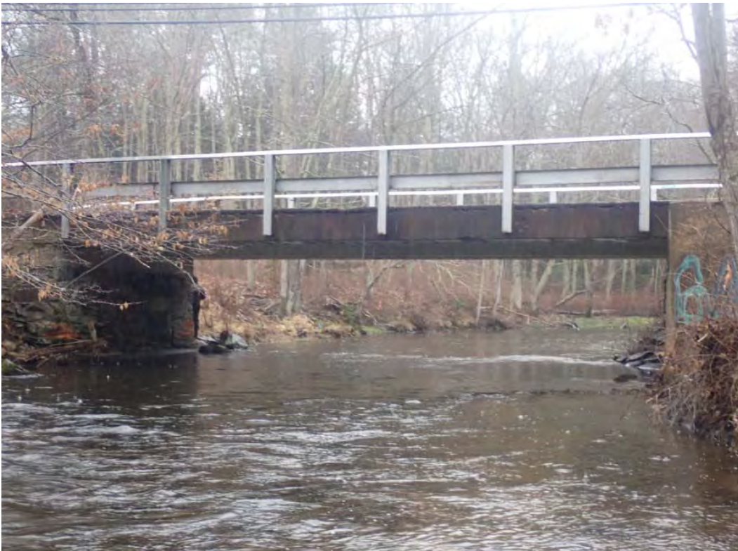
Image 2: South (downstream) face of Bridge #04730 looking northwest from the Fenton River.
