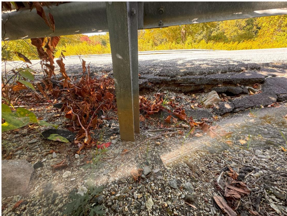
Typical View of Undermining at Shoulder (South East Corner Shown)
