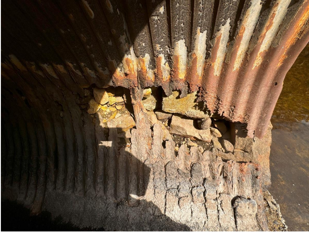
Typical View of Section Loss in Barrel (Barrel 1 Shown)
