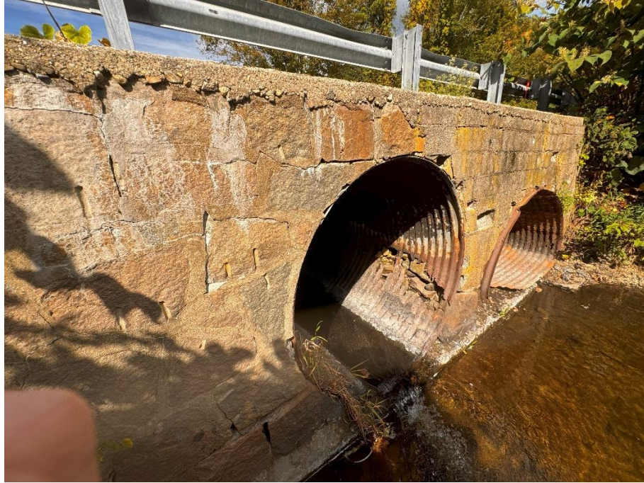
Headwall (down-stream)
