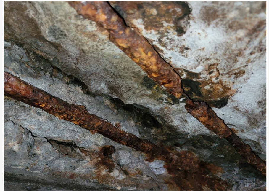
Heavy spall with rusted rebar with section loss
