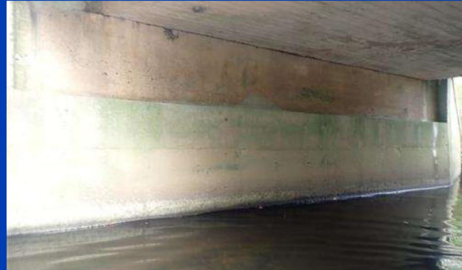
West abutment and underside of deck.
