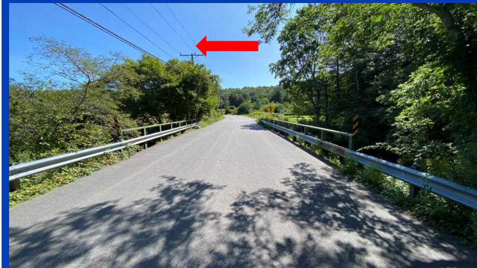
Bridge from west approach. Note: overhead utilities on north side of the bridge.
