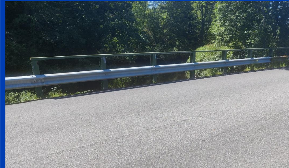
Bridge rail and overlay condition.
