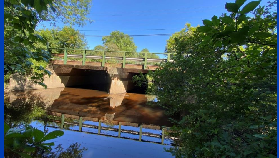
South (Downstream) Elevation
