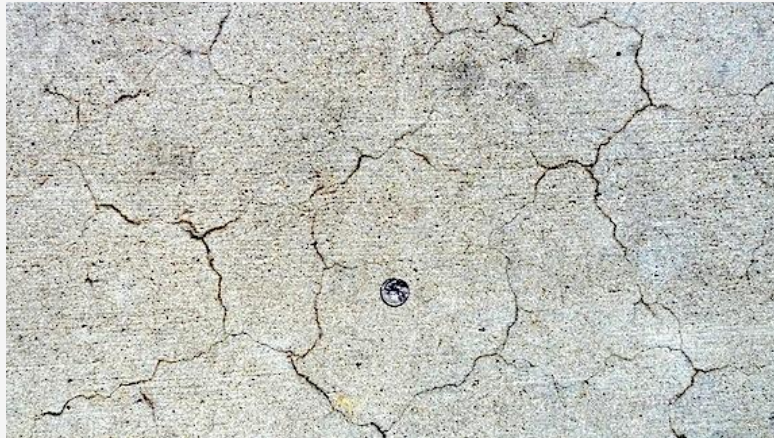
Map Cracking
