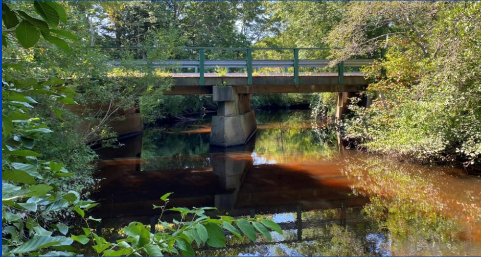
North (Upstream) Elevation
