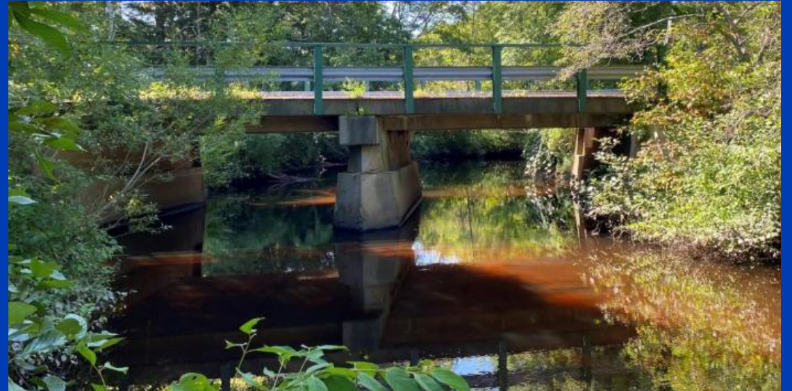
North (Upstream) Elevation
