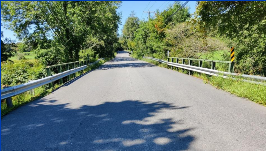
Bridge from east approach.
