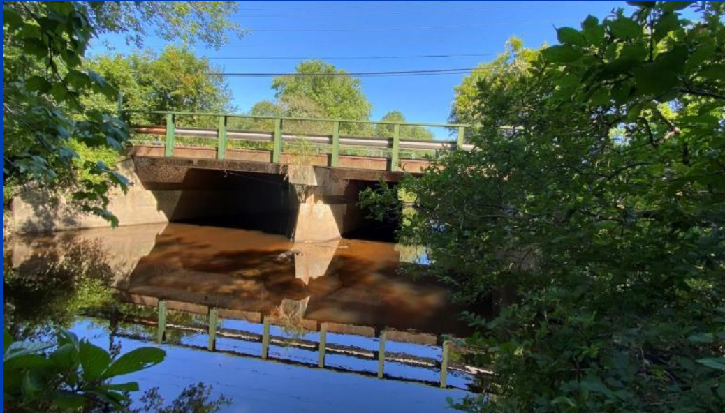
South Elevation View of Bridge
