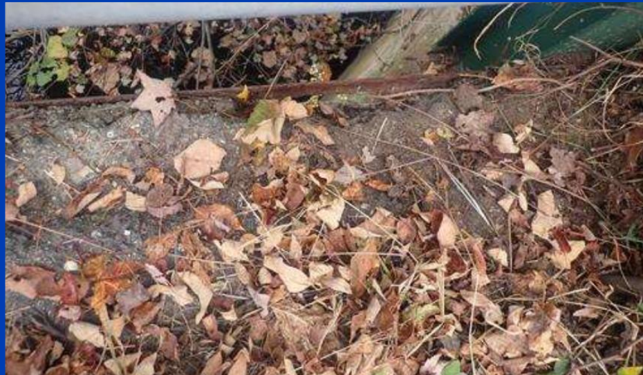
Deck spalling at the northeast fascia.
