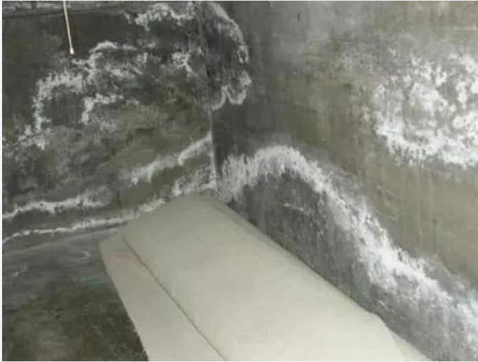
Efflorescence
