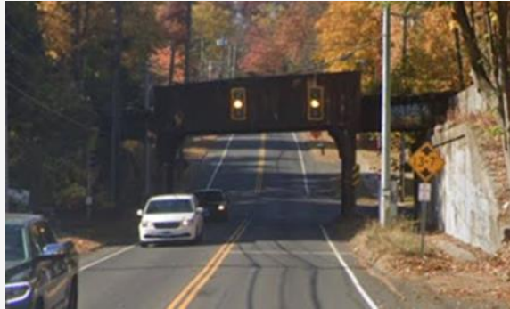
US Route 6 – East leg of the intersection (Looking West)
