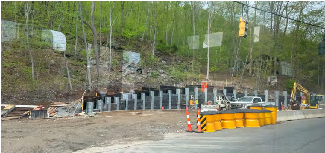
Figure 17. Topography requiring a retaining wall to install this roundabout, Higganum Village
