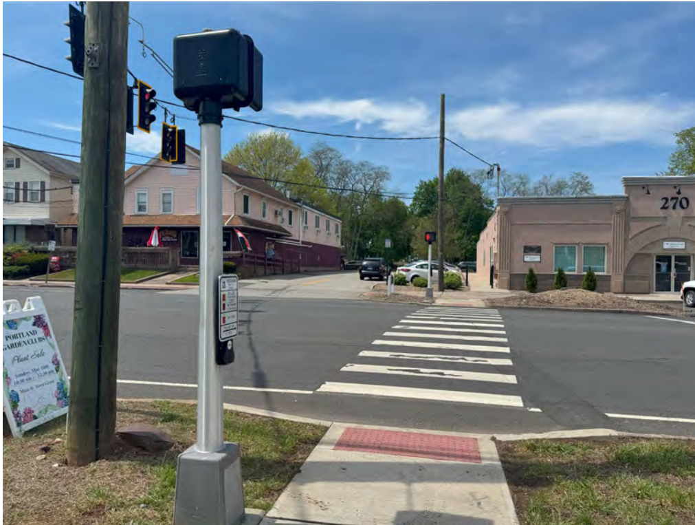
Figure 26. Pedestrian signal head with countdown timer, Portland
