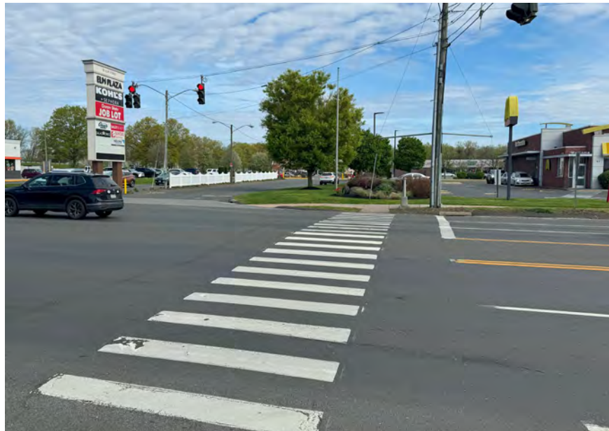
Figure 5. Intersection lacking pedestrian signal head and ADA compliance on Route 220, Enfield
