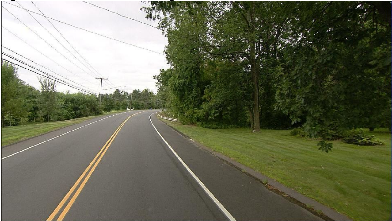
Figure 6. 3.0% RAS 1 Year Following Construction
