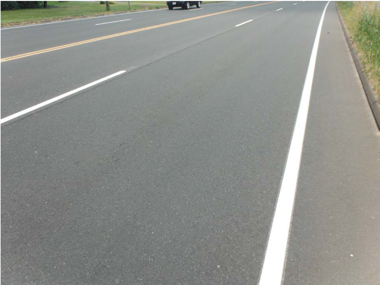
Figure 7. Rt. 220 HMA Control Section Summer 2014
