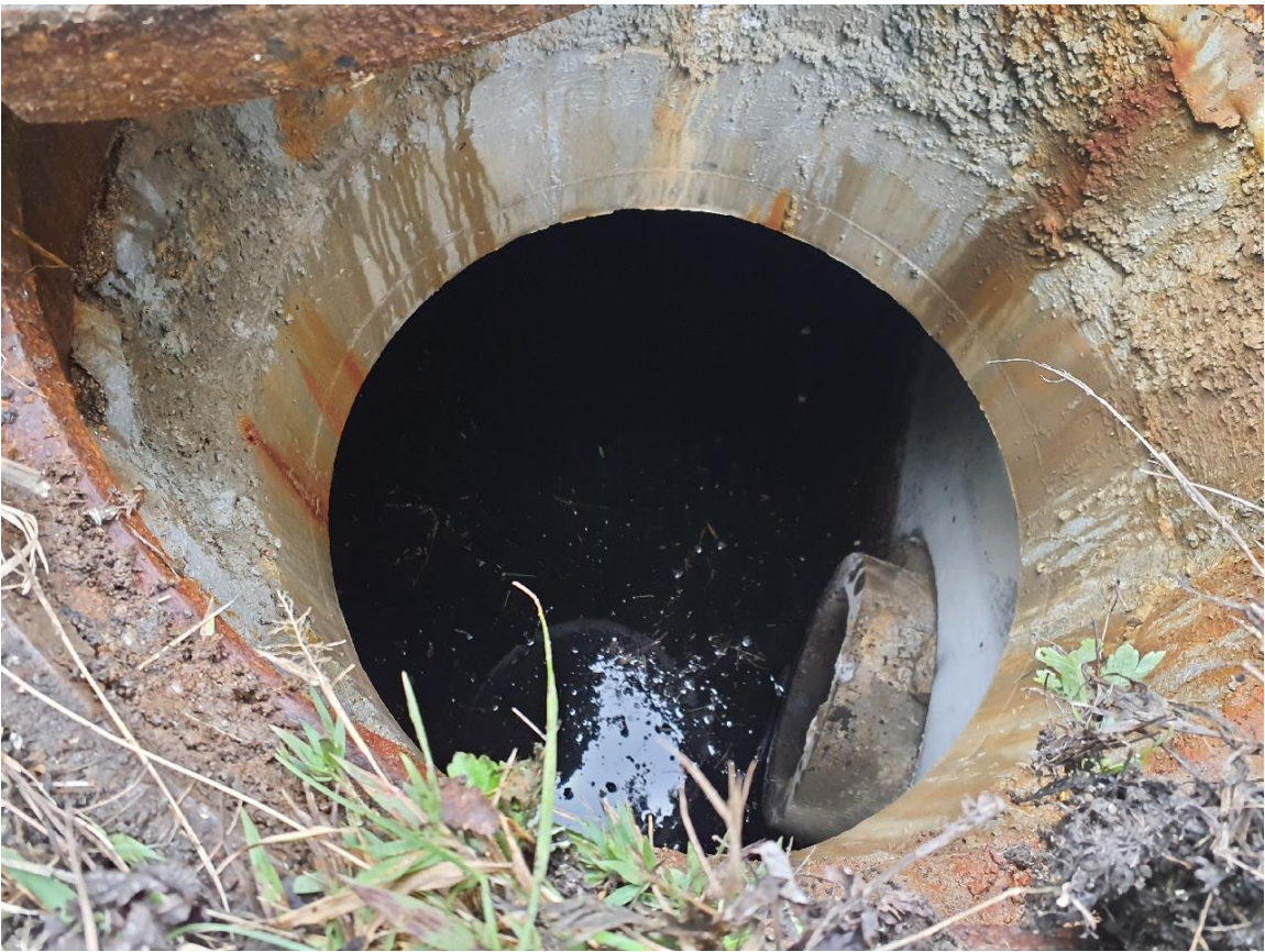
Underground detention system from above Image credit: Fuss & O'Neill
