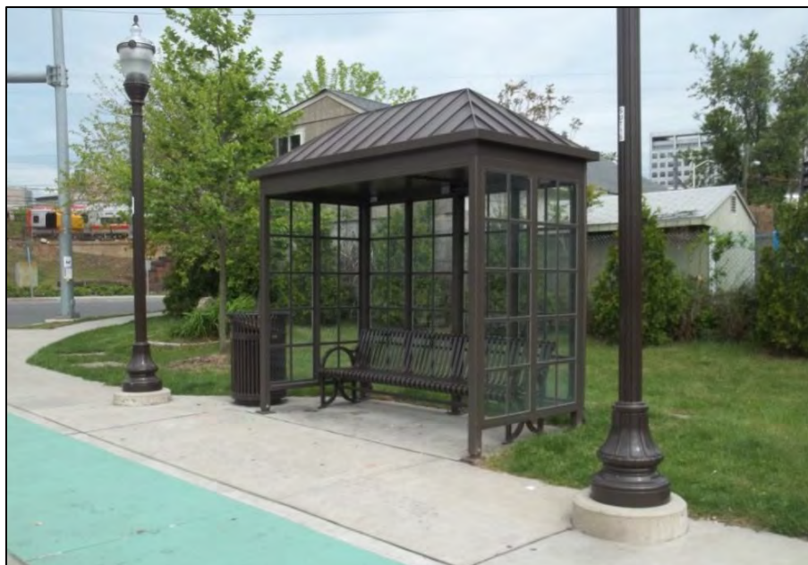
Exhibit 3-9: Bus Shelter at Dock Street & Atlantic Street
