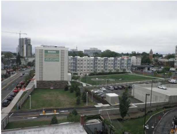
Exhibit 3-10: View looking south from Stamford Transportation Center Parking Garage, showing Metro Green Apartments (foreground) and Harbor Point development under construction (background).
