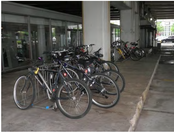
Exhibit 3-6: Existing Bike Racks under I-95
