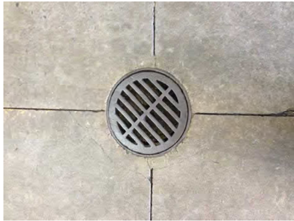
Photo 17: Representative floor drain inside building
