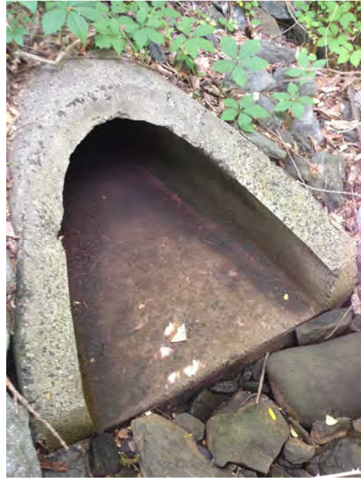
Photo 22: Close-up of drainage ditch from detention basin (facing northwest)
