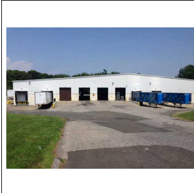
Photo 1: View of entrance to Site building (facing northeast)
