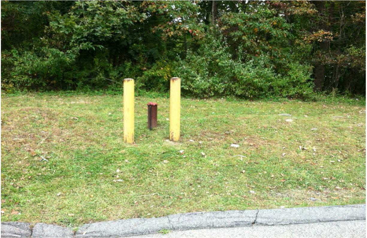
Water supply well located northwest of can recycling center building
