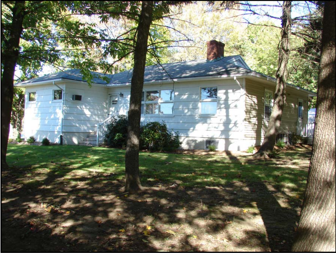
Photograph 3: House at 69 Marsh Hill Road, view northeast.
