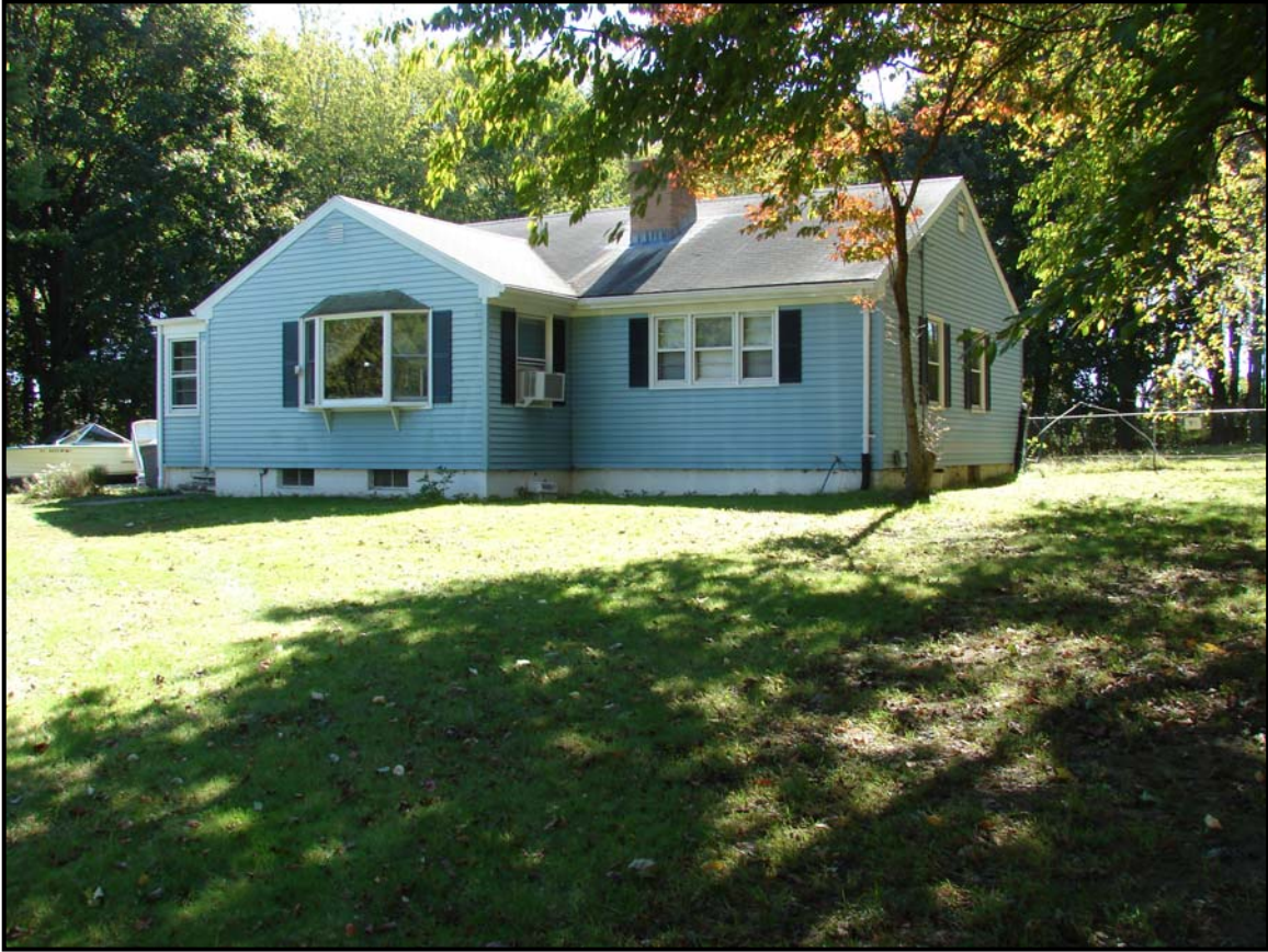
Photograph 1: House at 15 Salemm Lane, view southeast.
