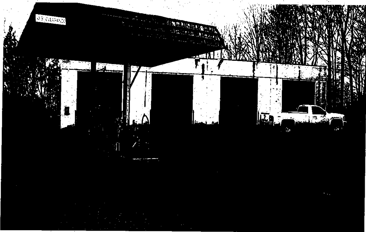
Photograph #4 - View of the repair garage and pump island, facing southwest.
