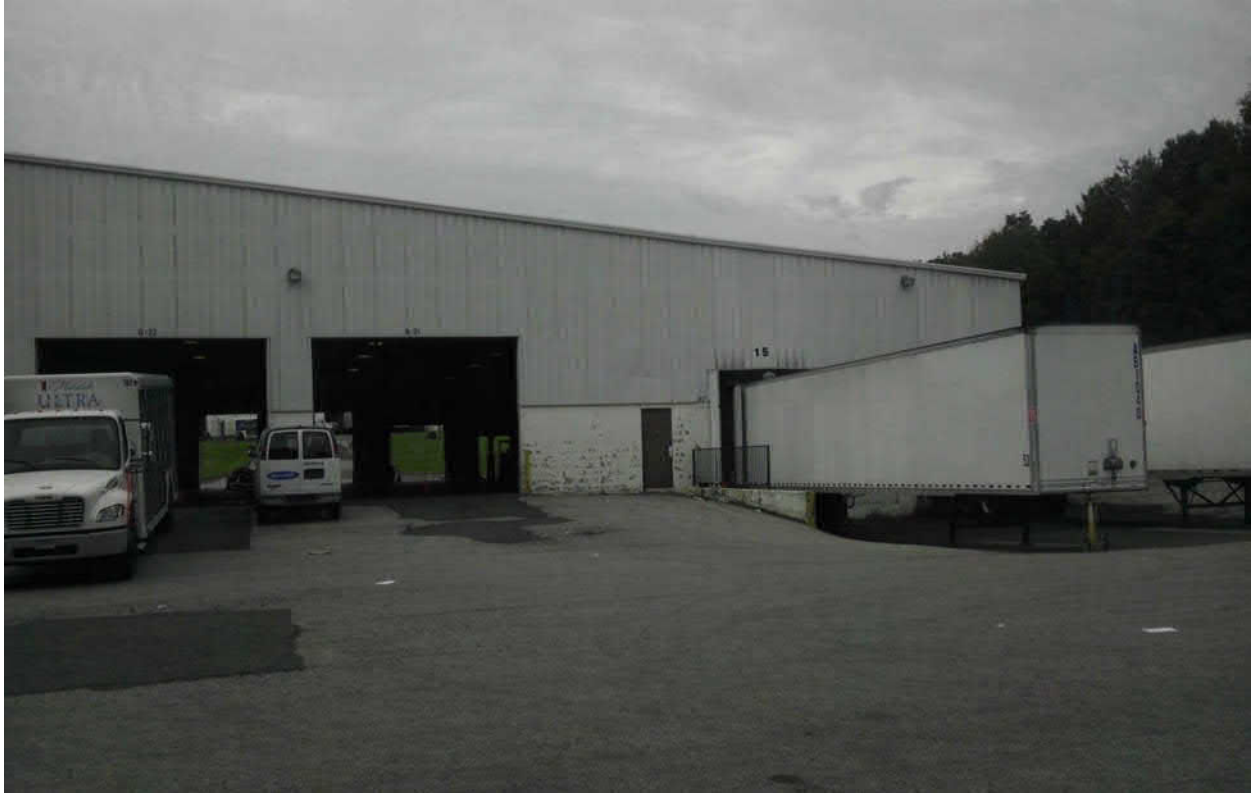
Loading docks, northeast side of can recycling center building
