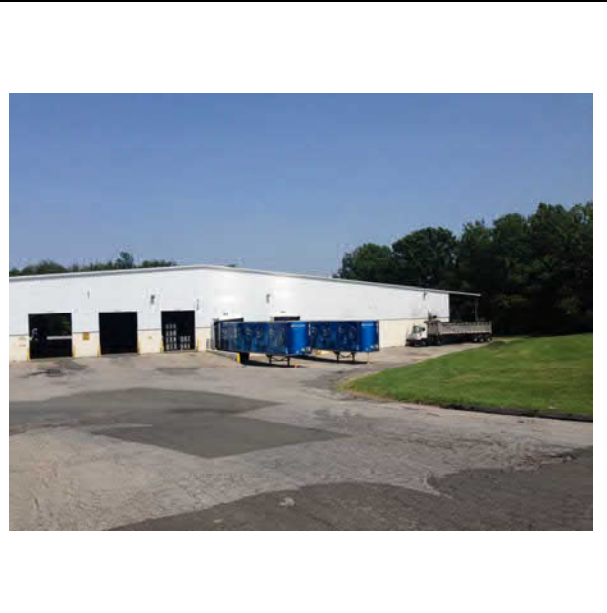
Photo 2: View of entrance to Site building (facing northeast)
