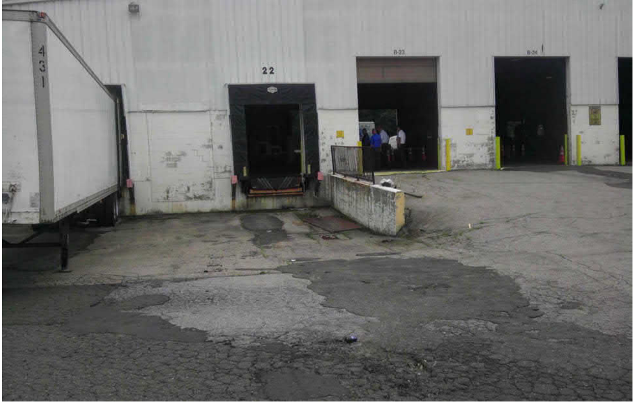
Loading docks, southwest side of can recycling center building
