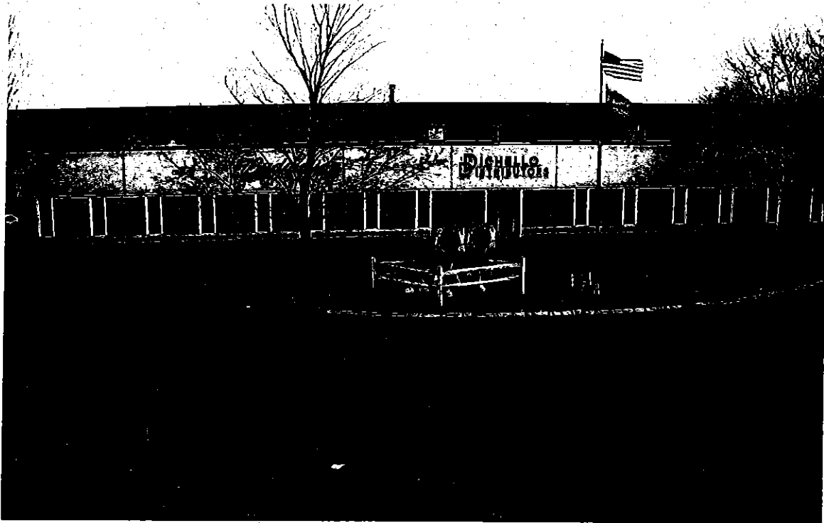
Photograph #1 - Front view of the distribution warehouse, facing southeast.
