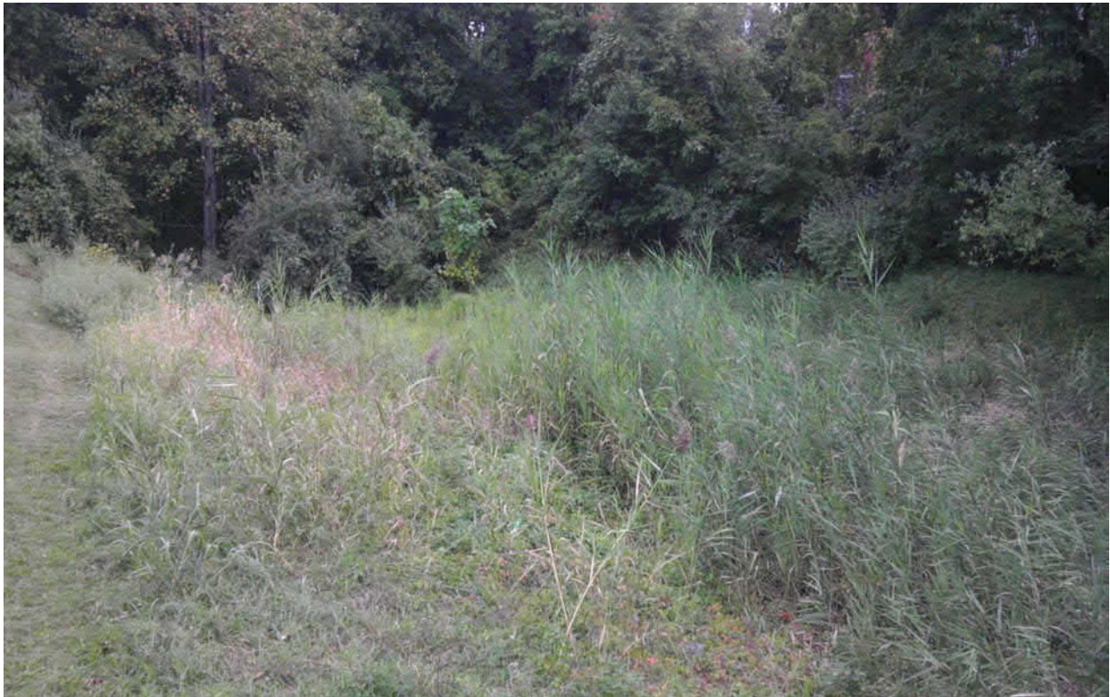
Detention basin located northeast of can recycling center building
