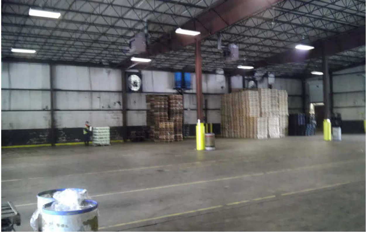
Northwest side of can recycling center building
