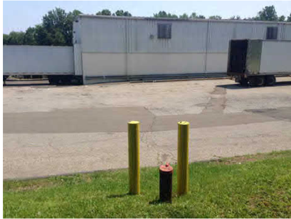
Photo 5: View of west side of building and bedrock water supply well (facing southeast)
