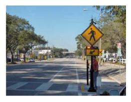
The RRFB is composed of amber light emitting diodes (LEDs) that supplement warning signs at uncontrolled approaches to unsignalized intersections or mid-block crosswalks. RRFBs use an irregular flash pattern that is similar to emergency flashers on police vehicles. RRFBs can be activated by pedestrians manually by a push button or passively by a pedestrian detection system.
