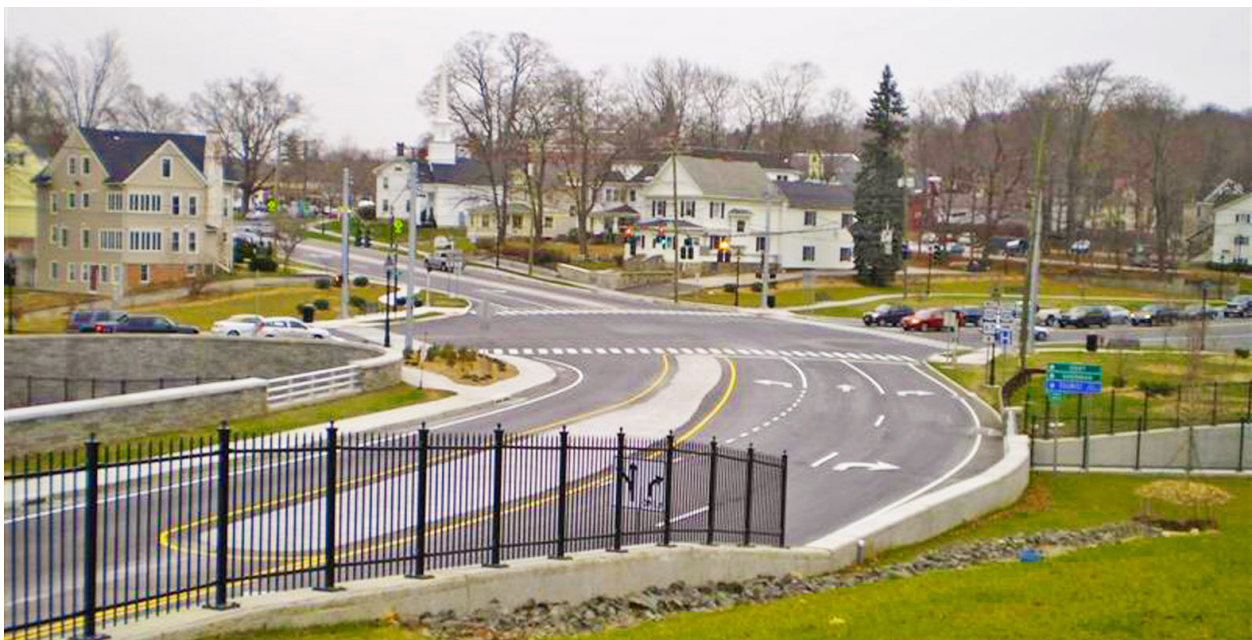
Figure 3.1: Route 67 and Grove Street Construction in New Milford.
