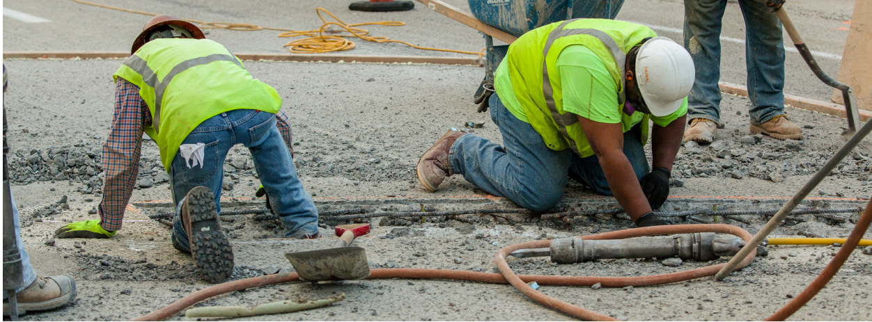
Figure 3.3: Workers performing resurfacing for bridge safety improvements on Route 2.
