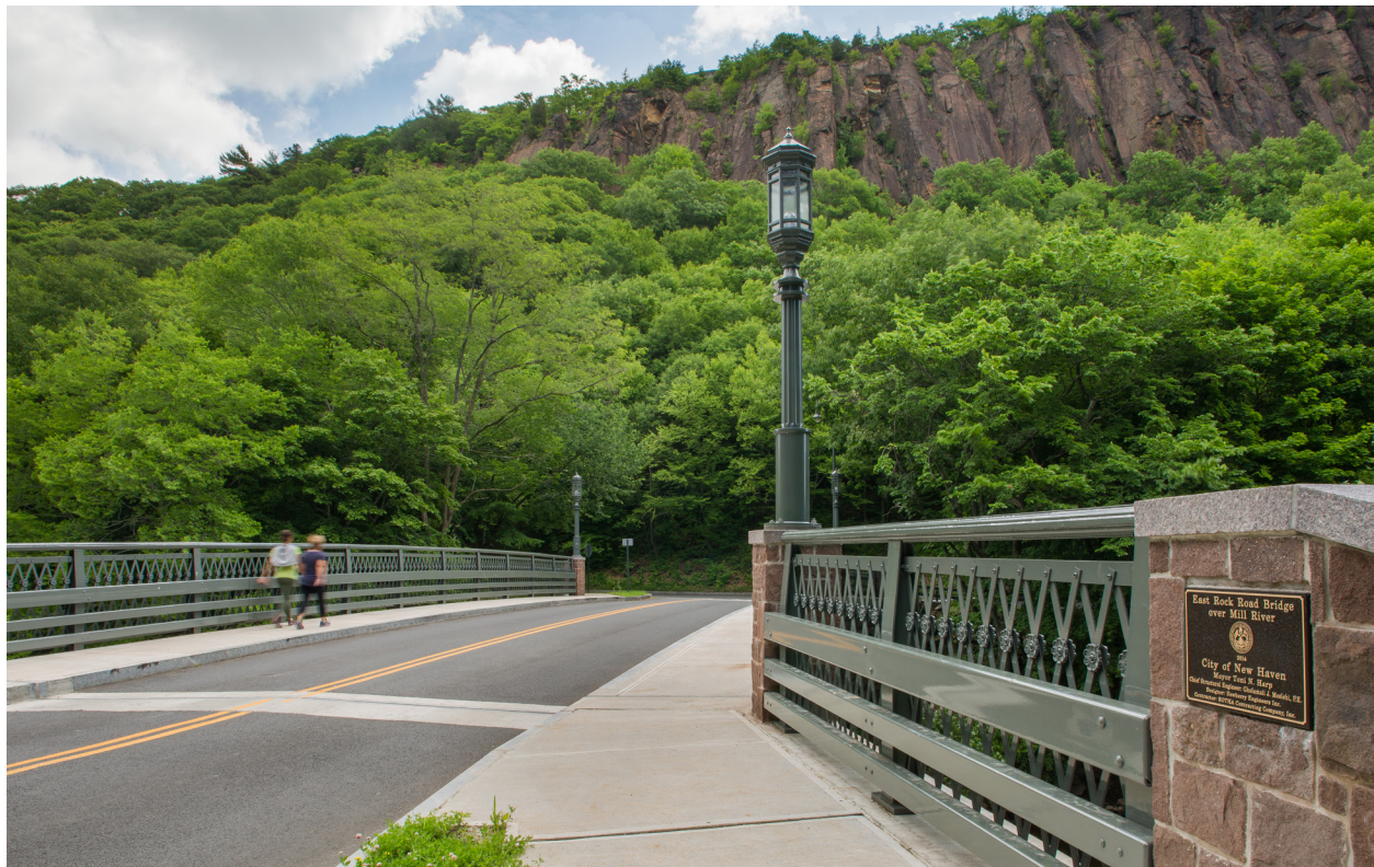
Figure 4.2: East Rock Road Bridge over the Mill River in New Haven.
