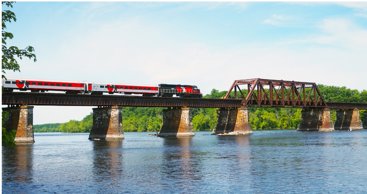
Figure 2.2: CTrail Hartford Line train across the Connecticut River Bridge.
