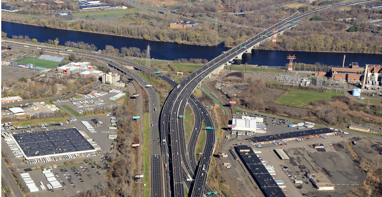
Figure 3.4: Aerial view of the I-91 Charter Oak Bridge Project.
