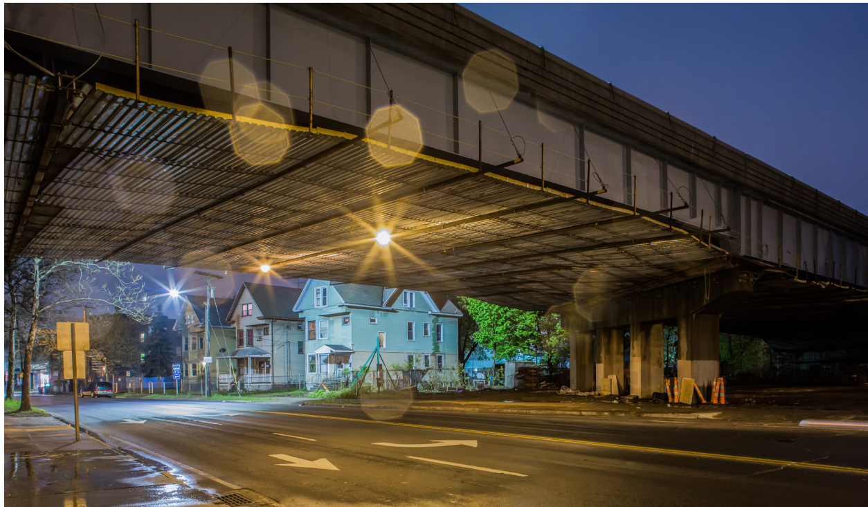
Figure 3.8: I-91 Bridge over Ferry Street in New Haven.
