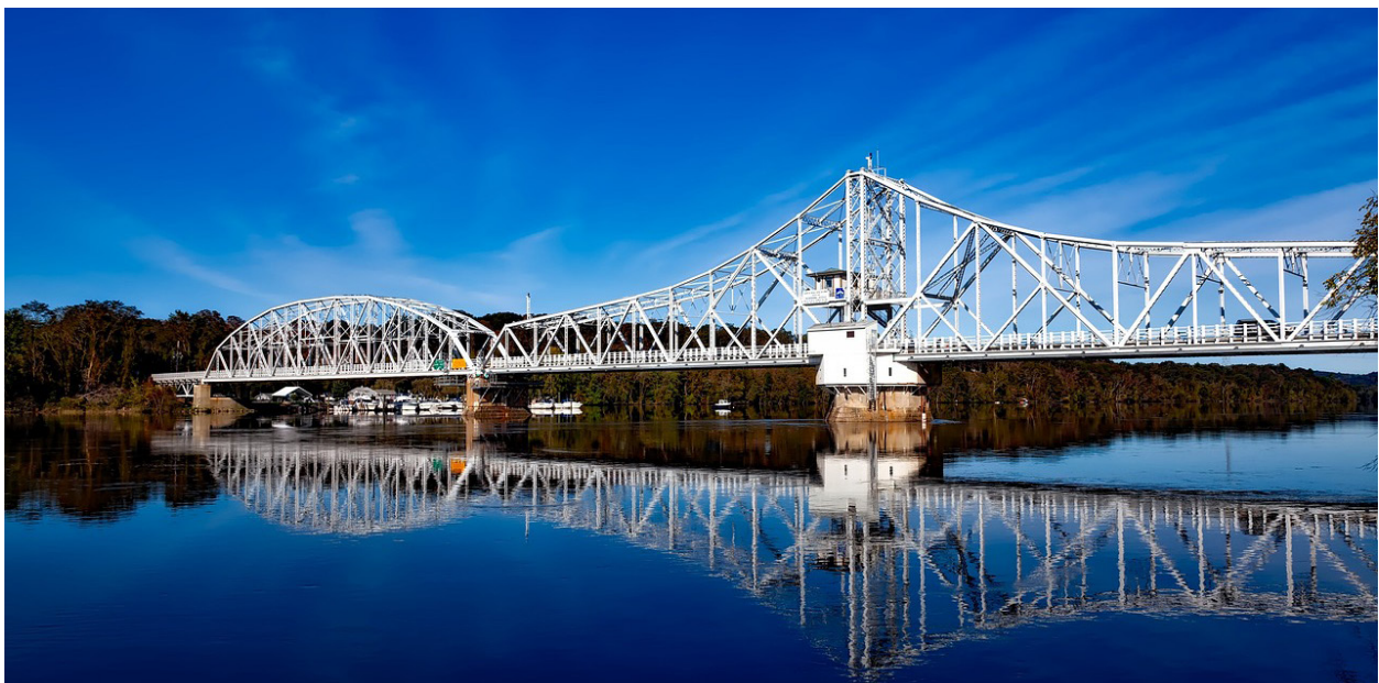
Figure 1.1: The East Haddam Swing Bridge over the Connecticut River.
