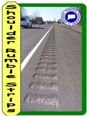
TRB Paper No. 05-1299, "Evaluation of Safety Benefits and Potential Crash Migration Due to Shoulder Rumble Strip Installation on Freeways in Connecticut"
