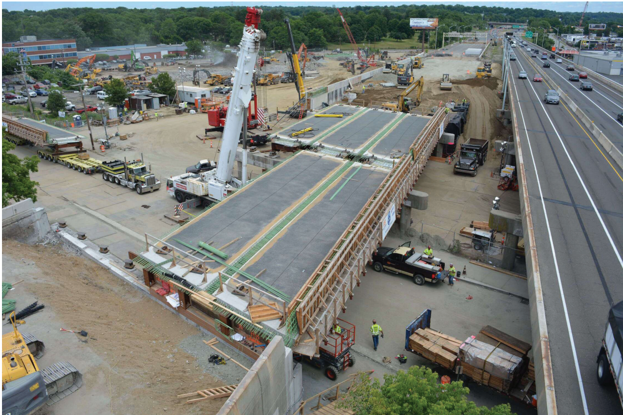
BRIDGEPORT DESIGN-BUILD PROJECT UNDER CONSTRUCTION (PHOTO COURTESY OF CTDOT)
