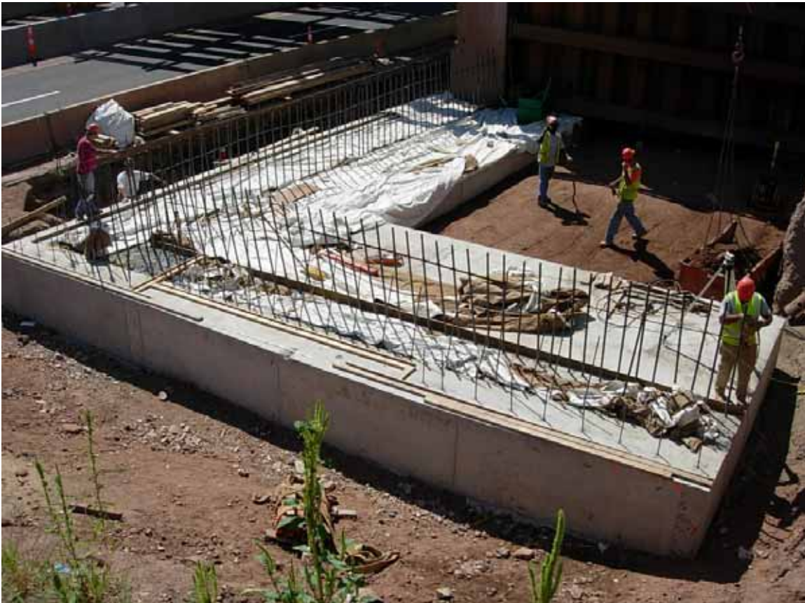
Figure 59 Bridge 1629 Stage 2 Footing for Abutment 2/Wingwall 2B.
