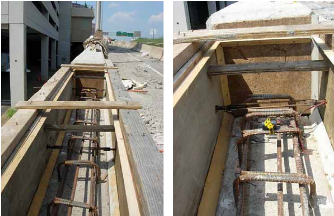
Figure 48 August 4 th Pour at Project 63-579 in Hartford
