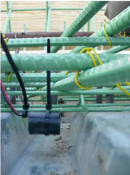
Figure 56 Probes installed in deck at top and bottom.
