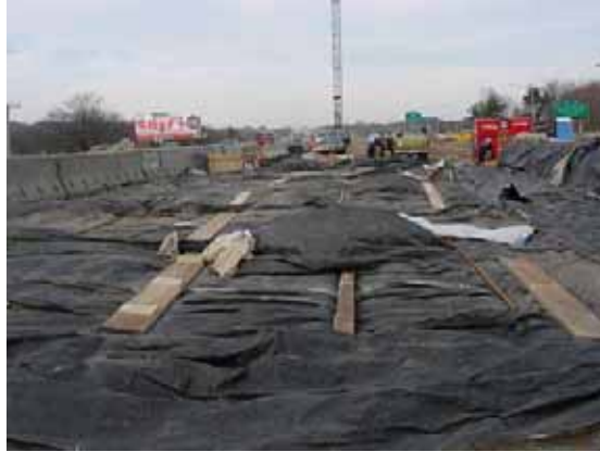
Figure 55 Bridge 182 SB Deck. Hot water hoses over rebar (left), and then covered in blankets (right).
