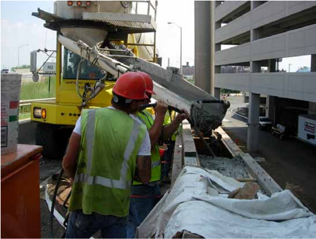
Figure 42 Hot-Weather Concreting at Project 63-595.
