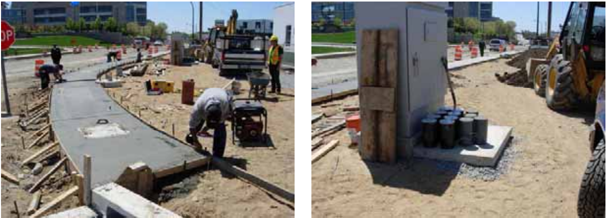
Figure 31 Concrete for sidewalk and 6"x12" specimens.
