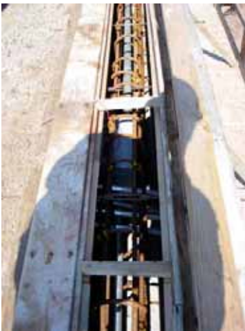
Figure 29 IntelliRock™ probe installed in Class "A" Modified concrete for Bridge 181 WW 2A parapet sections (2 nd and 4 th ).
