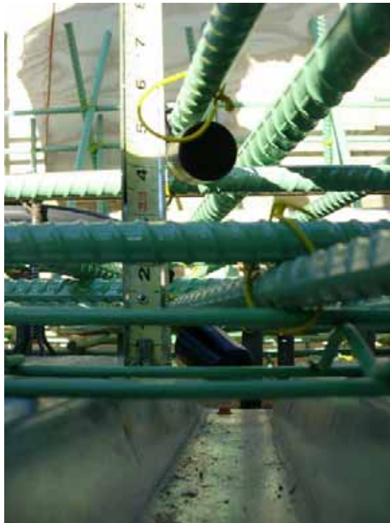
Figure 56 Probes installed in deck at top and bottom.
