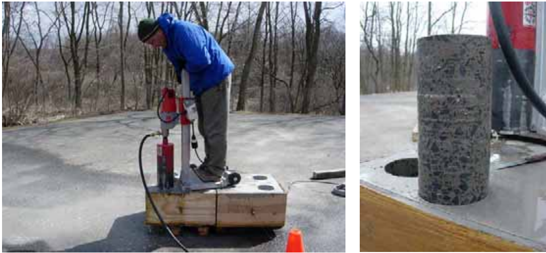
Figure 33 Obtaining drilled cores from concrete blocks.
