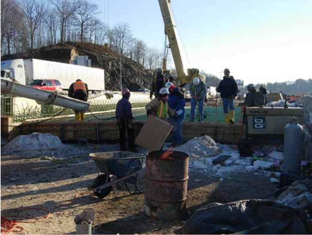
Figure 50 Cold-Weather concreting at Project 43-122.
