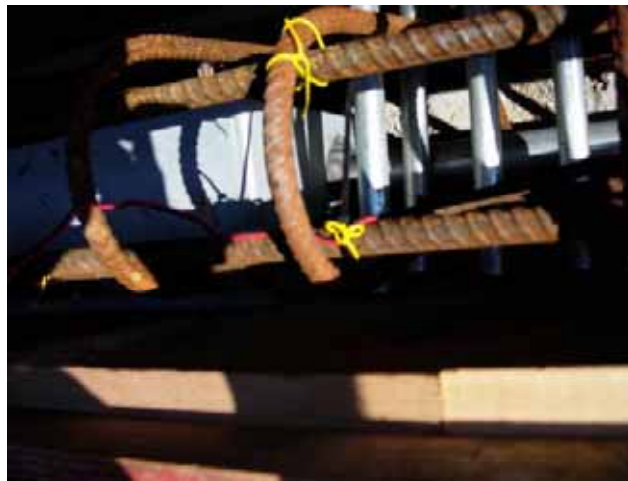
Figure 29 IntelliRock™ probe installed in Class "A" Modified concrete for Bridge 181 WW 2A parapet sections (2 nd and 4 th ).
