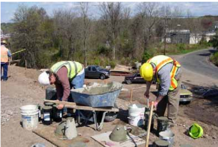
Figure 30 Research staff testing concrete side-by-side with consultant inspector at Project 43-122.
