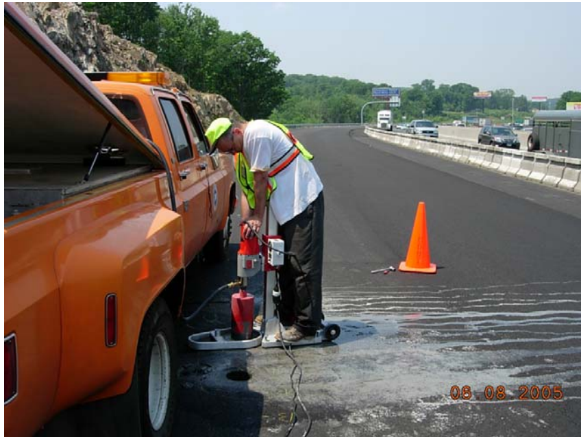
Photo #6, ConnDOT Portable Coring Rig Cutting Cores on I-84
