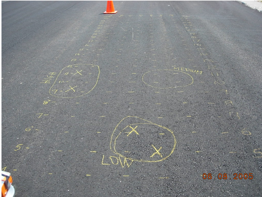
Photo #7, Coring and Measurement Grid, I-84
