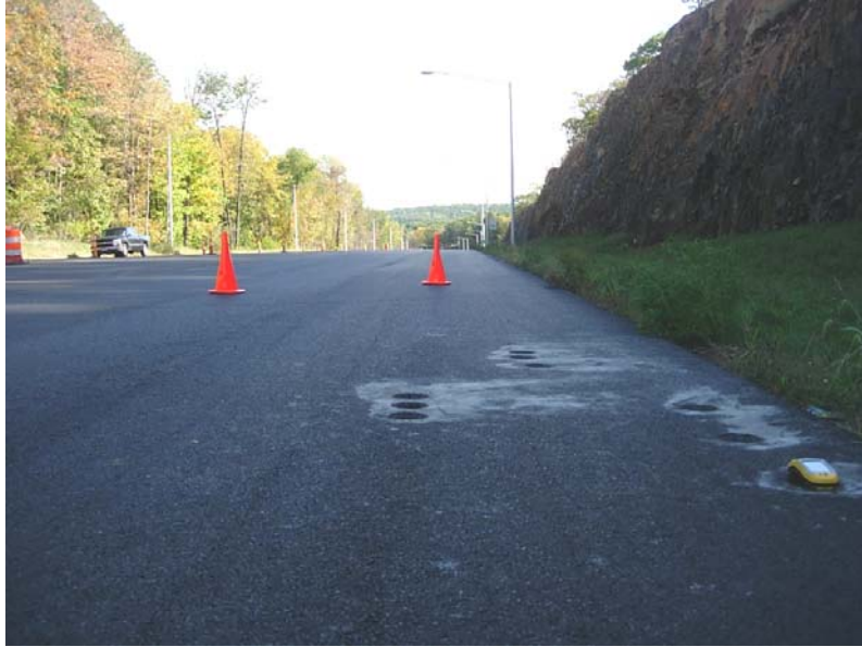
Photo #11 Cores Removed Route 66, Middlefield
