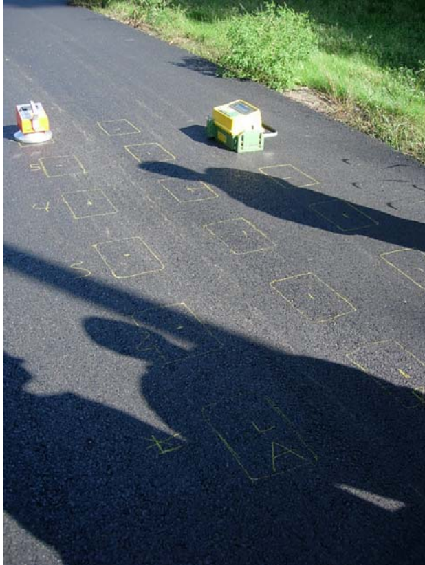
Photo #9, Coring and Measurement Grid, Route 66
