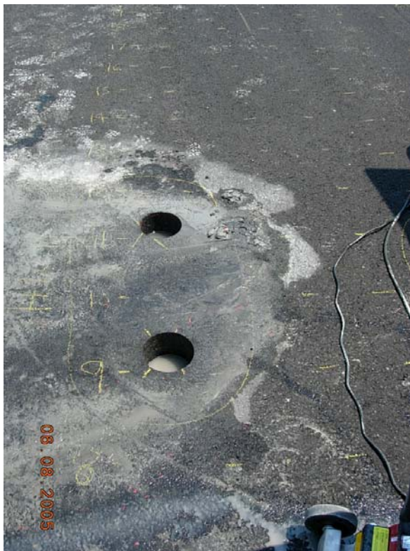
Photo #10, Cores Removed (A9, B11), Route I-84
