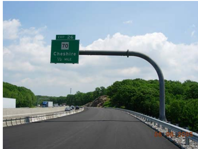
Photo #1, I-84 Eastbound, Waterbury (Project 151-274)
