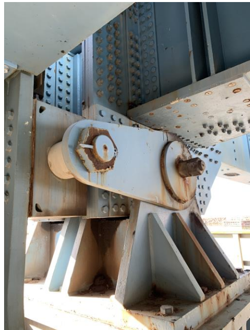
Lift span fixed bearing
