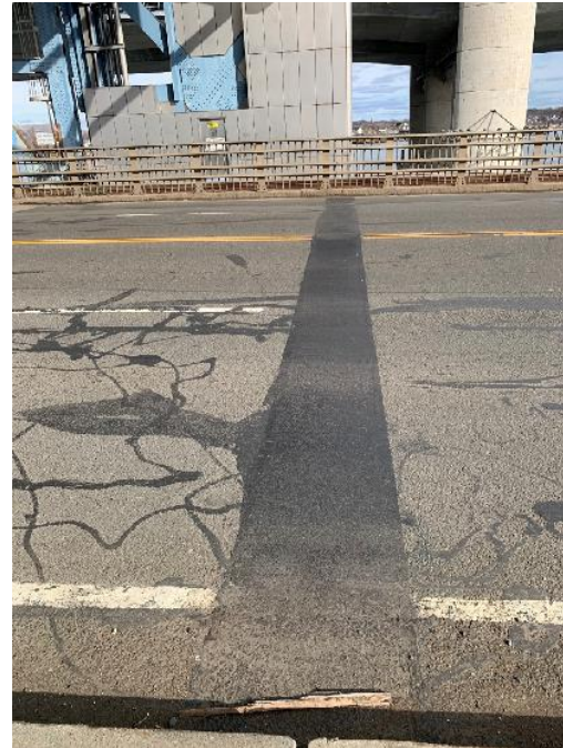
Asphaltic Plug Joint (Typ.)
