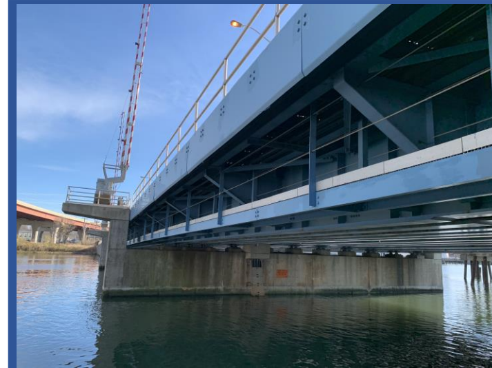
Pier typical condition (Pier 2E).
