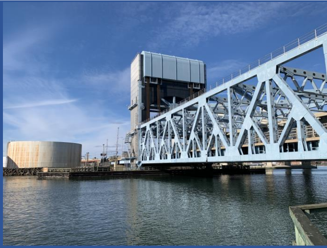
Channel under bridge, looking Northwest.
