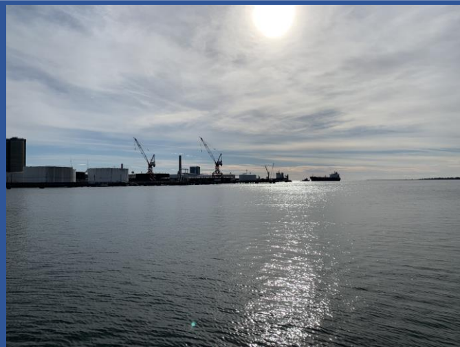
Channel downstream of bridge (New Haven Harbor/Long Island Sound), looking Southeast.
