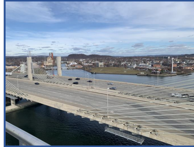
Channel upstream of bridge (Quinnipiac River), looking Northwest.
