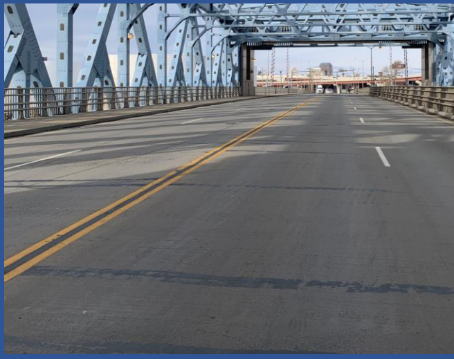
Top of Bridge at Lift Span (Looking West)
