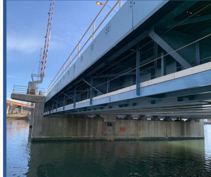
Typical Approach Span Elevation
