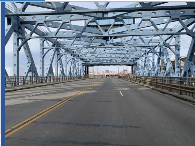
Through view of lift span, looking west.
