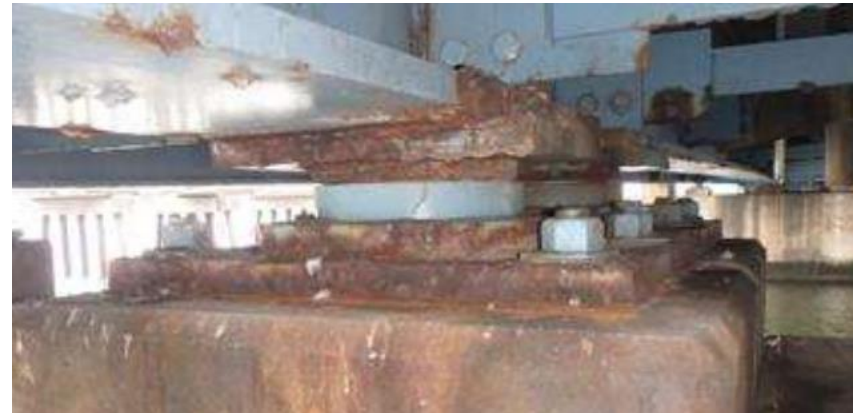
Typical Approach Span Bearing
