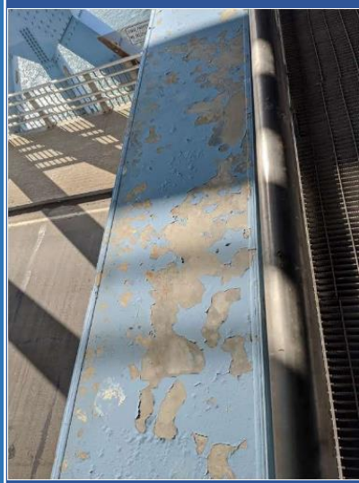
Peeling paint on lift span fascia bracing.
