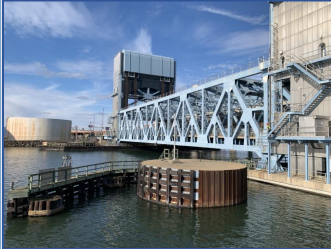
South Fascia of lift span, looking northwest.
