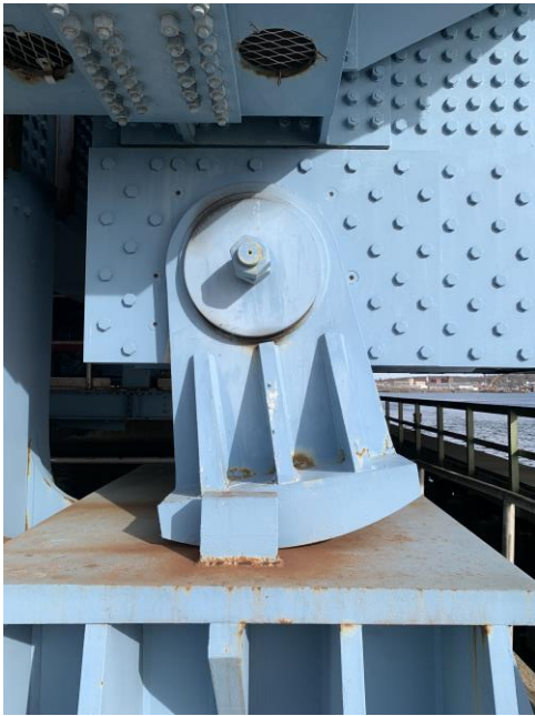
Lift span expansion bearing in fully expanded position
