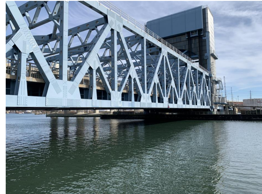
Rehabilitation of Bridge No. 00337 // State Project No. 0092-0687
