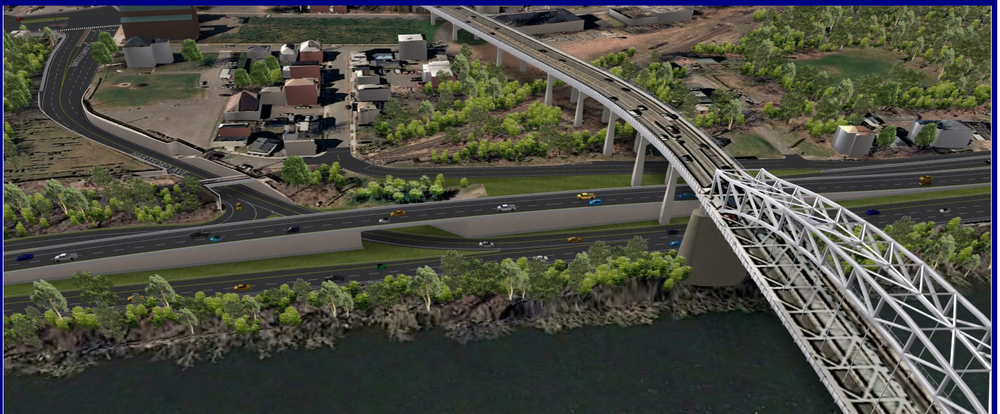
FIGURE 1—ROUTE 9 SOUTHBOUND OVER THE HARTFORD AVENUE ROUTE 9 NORTHBOUND ON-RAMP
