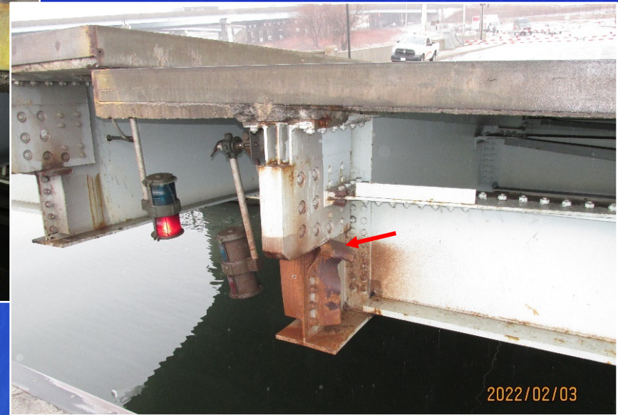
Diaphragm with Bent Live Load Shoe
