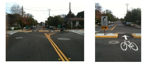
**Pros** :: Reduces cut-through traffic; Channels traffic flow, thus eliminating vehicular conflicts at some intersections; can be designed to accommodate emergency
