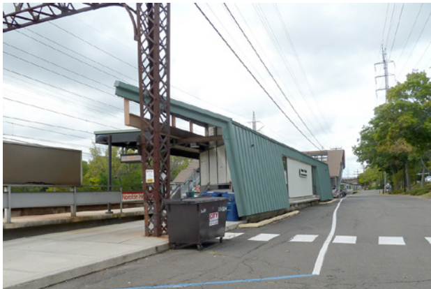
Figure 9: Photo of the station building and its lean-to canopy
