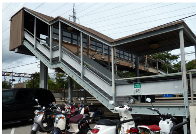
Figure 11: Photo of the pedestrian bridge connecting the two platforms
