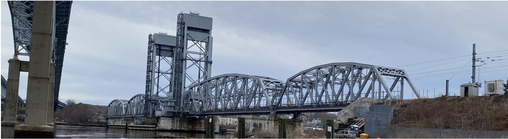
Thames River Moveable Bridge
