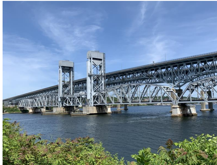
Thames River Moveable Bridge
