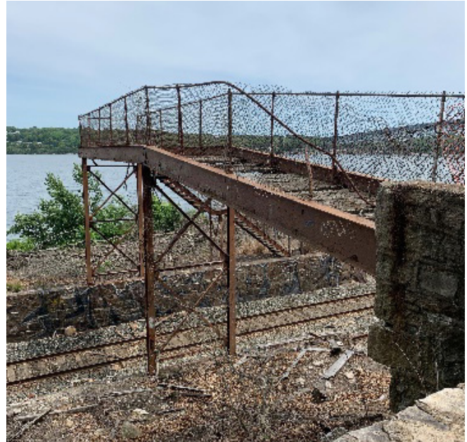
Figure 13 Abandoned Bridge at Riverside Park
