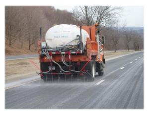
The Department pre-treats certain highways and bridge decks with a 23 percent solution of sodium chloride brine (salt brine) throughout the winter season to mitigate the bond of snow and ice to the pavement surface. The pre-treatment is performed at locations that have a tendency for frost formation and prior to winter storm events.
