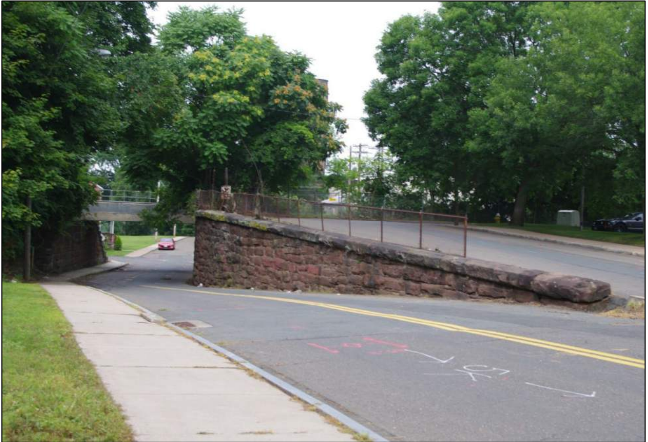
Image 1: Retaining wall (ca. 1900) adjacent to Main Street underpass, camera facing west.
