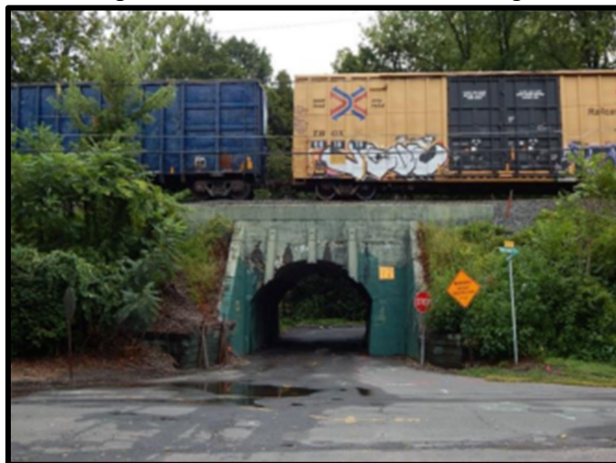
Figure 2-5: West Portal of Asnuntuck Bridge
