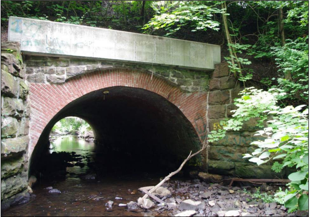
Image 3: Freshwater Brook Railroad Bridge, east elevation, camera facing northwest.
