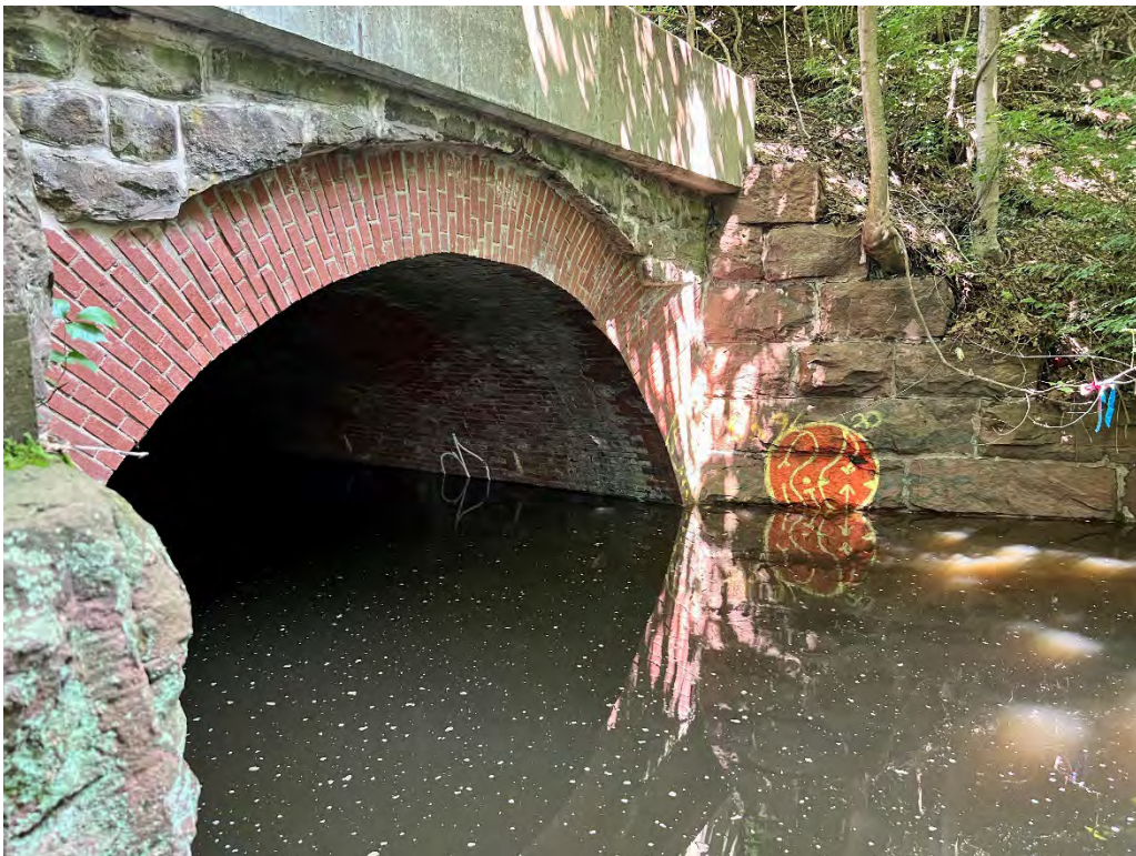
Freshwater Brook bridge under rail line (July 2023)
