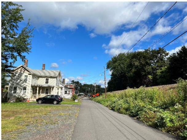
5. The rail corridor (at right) is elevated and visually prominent in the Study Area.
