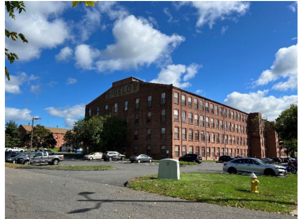
2. One of several Bigelow Commons residential buildings, looking northeast from the Project Site.
