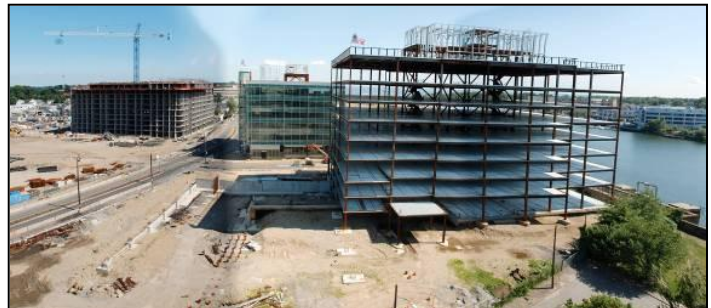
Construction at Harbor Point.
