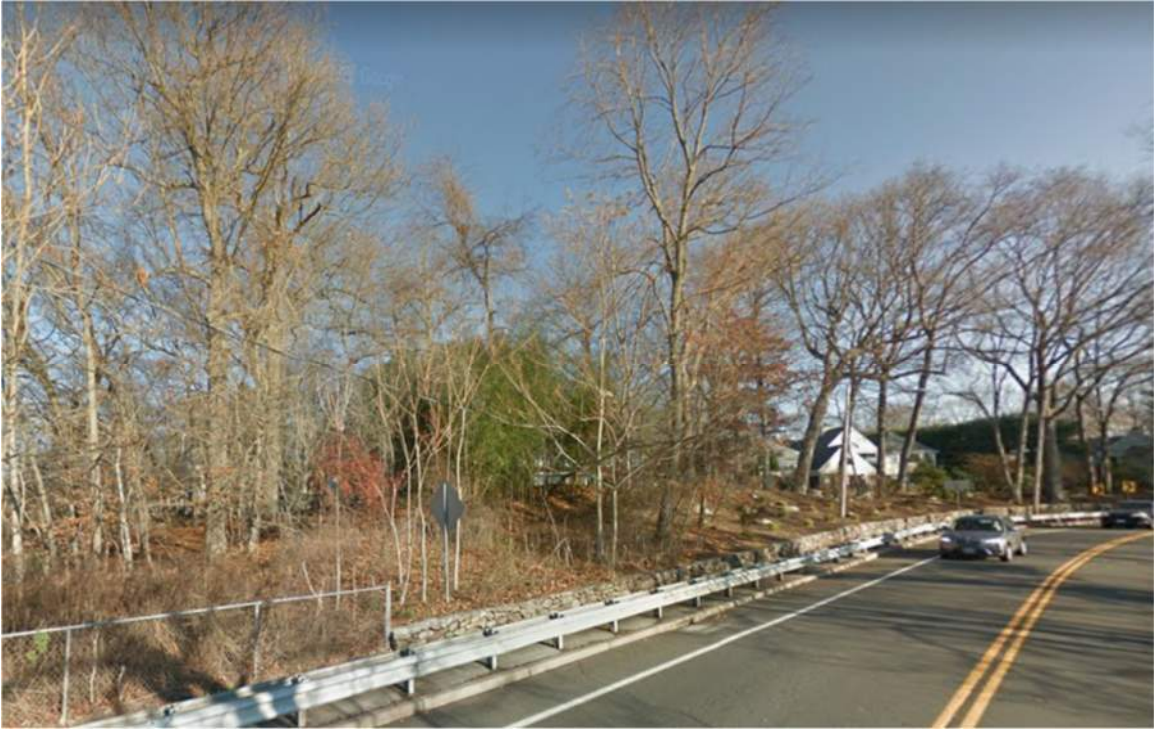
Image 7: Western terminus of stone wall that abuts the property at 5 Imperial Landing. The wall is within the existing road right of way.
