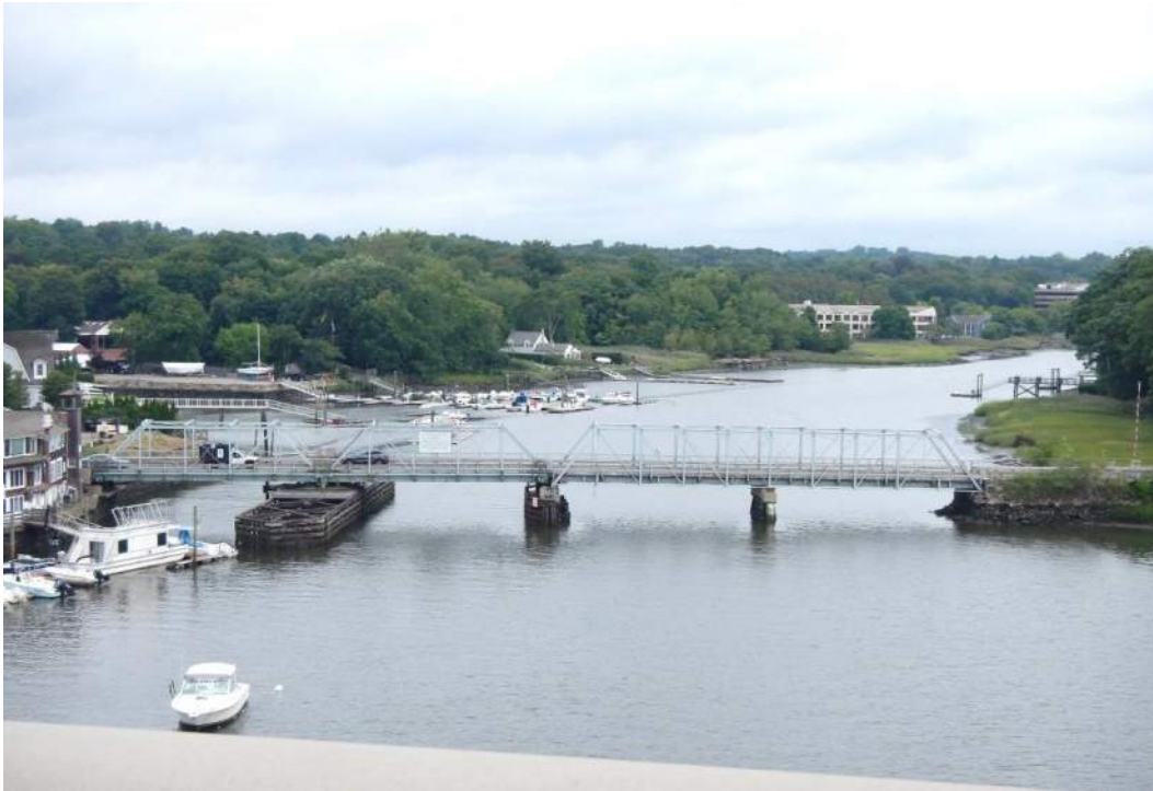
Image 1: Southern face of Bridge #01349, viewed from I-95.
