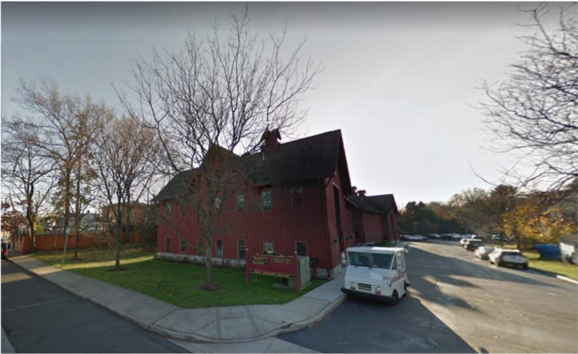
Image 10: Old barns at 518 Riverside Avenue.
