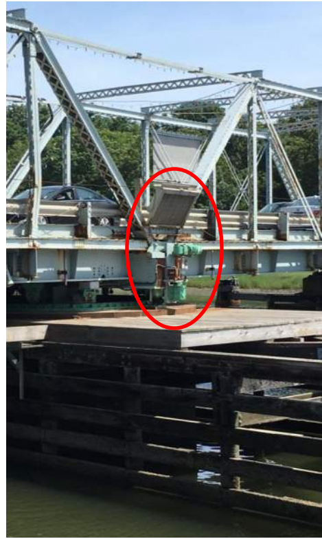
Image 12: The south side of the swing span now features an electric motor at the screw jacks (left photo) and at the center of the swing span (right photo, outlined) that are responsible for opening and closing the span. This is a minor change in the appearance of the bridge.
