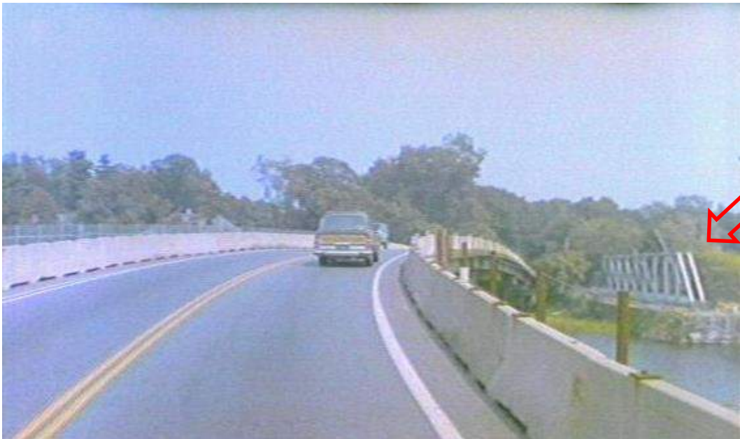
Image 5: View of Bridge #01349 from the temporary bridge installed to carry Route 136 during the 1991 rehabilitation. Note that the trusses have been moved from their original locations intact and are staged on the approach roadway (red arrow).
