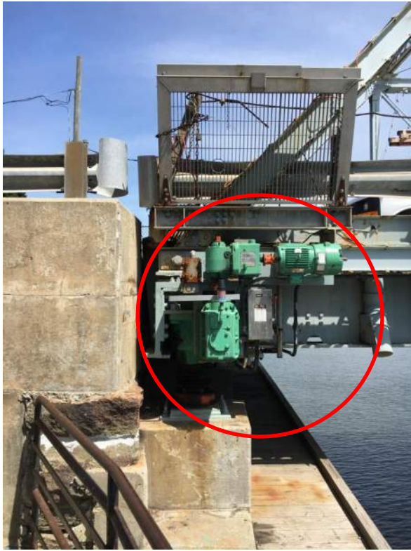
Image 12: The south side of the swing span now features an electric motor at the screw jacks (left photo) and at the center of the swing span (right photo, outlined) that are responsible for opening and closing the span. This is a minor change in the appearance of the bridge.
