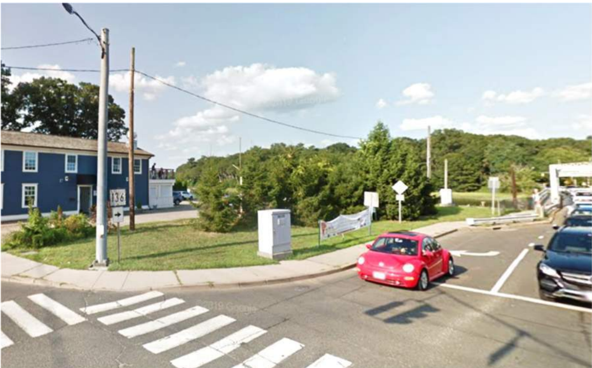
Image 8: Block 59 / Lot 000 (grass covered area) at the northwest corner of Bridge #01349. This property is owned by CTDOT and served as the approach for the detour bridge that was required for the previous rehabilitatoin in 1991.
