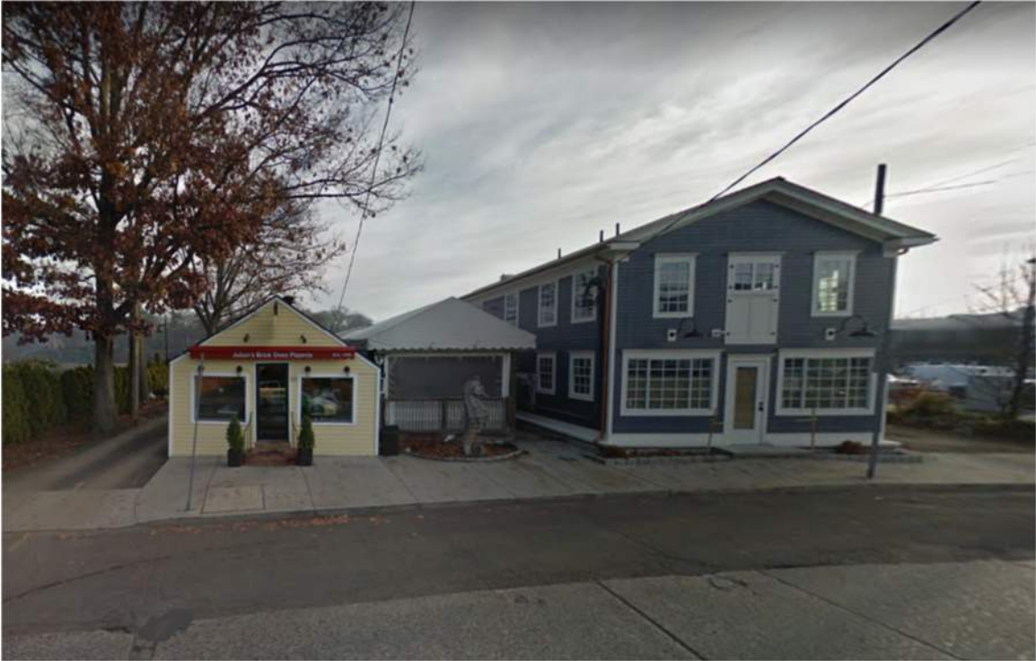
Image 13: Restaurants at 535 Riverside Avenue. Each building was originally constructed as part of the Rufus Wakeman Mattress Factory.
