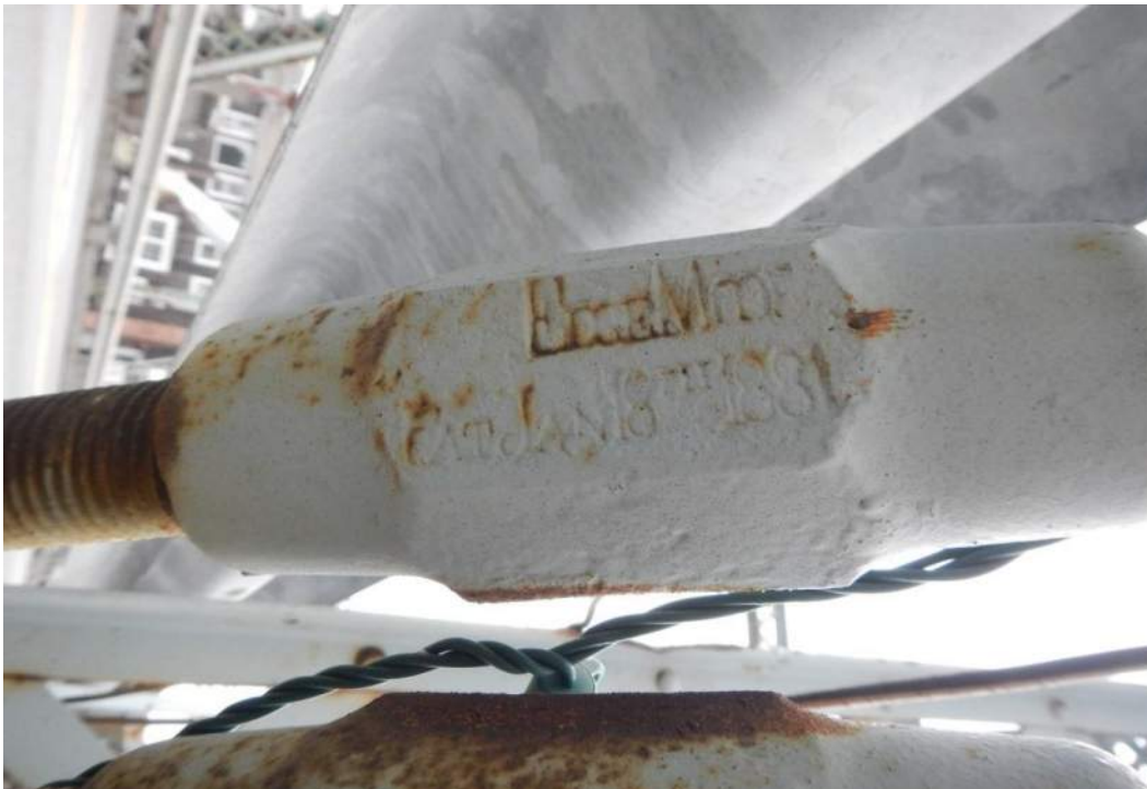
Image 7: Cast iron turnbuckle bearing the label “EdgeMoor – Pat [Patent] Jan 18 th 1881”
