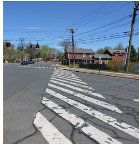
Figure 14. Long, Skewed Crossing at Deerfield Road
