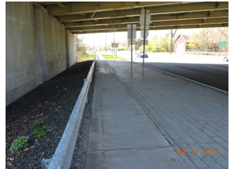
Figure 11. Lack of Lighting Under the Overpass Bridge
