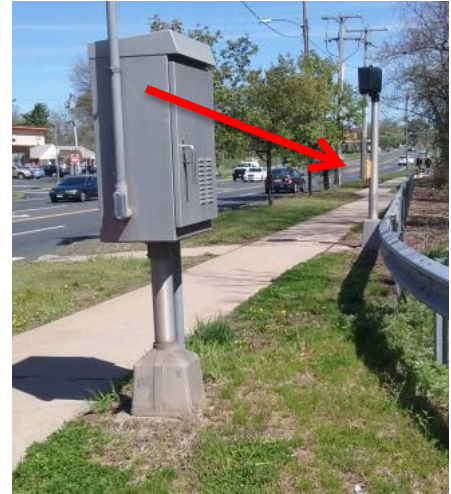
Figure 10. Pedestrian Push Button Far From Crosswalk
