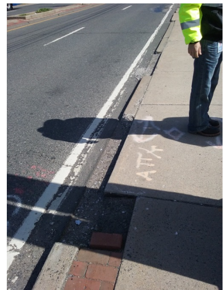
Figure 6. Broken Curbing
