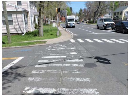
Figure 18. Loop Detectors Within Crosswalk
