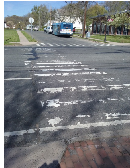
Figure 9. Faded Crosswalk
