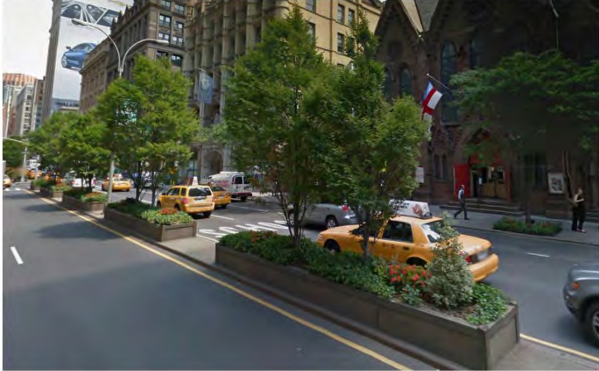
Exhibit 53: An example of landscaping in a narrow, raised median on Park Avenue South in New York, NY (Source: NYCDOT)
