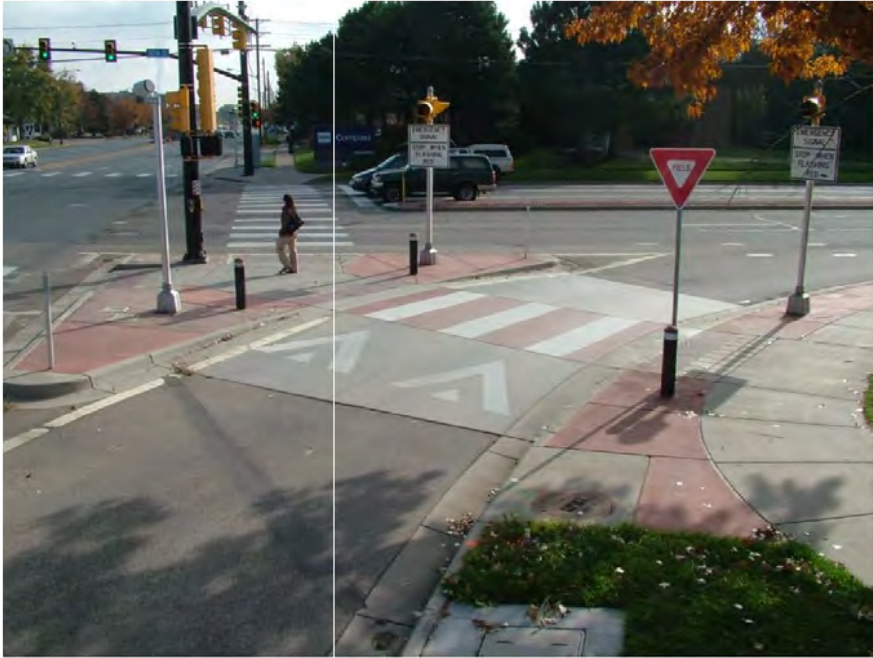
Exhibit 48: Channelized right-turn lane with raised crosswalk in Boulder, Colorado (Reference: NCHRP 208, Design Guidance for Channelized Right-Turn Lanes (2014))
