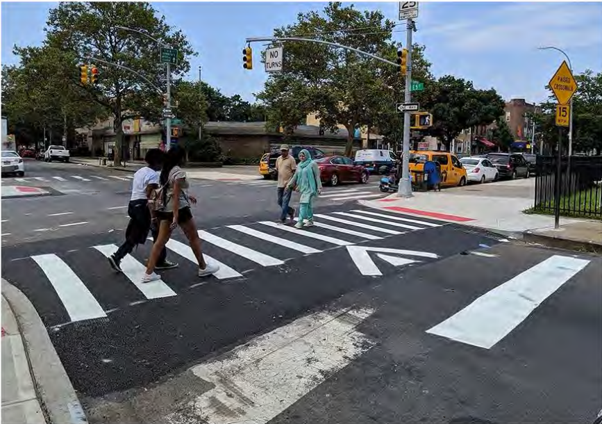
Exhibit 55: A raised crosswalk across a side street intersection (Source: NYCDOT)
