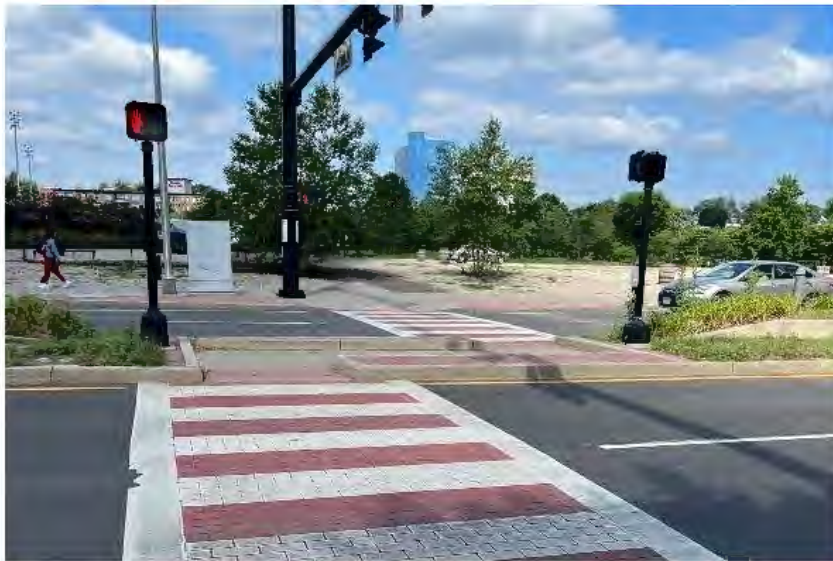
Exhibit 37: The Pedestrian Hybrid Beacon (or "HAWK") in front of Mill River Park
