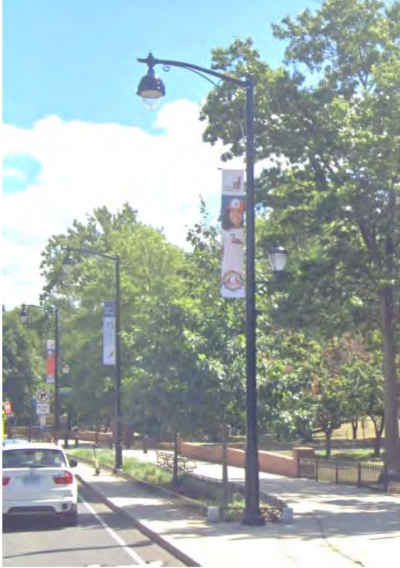
Exhibit 54: Street light with both traffic-side and sidewalk-side luminaire in Hartford, CT. (Source: Google Earth Streetview)
