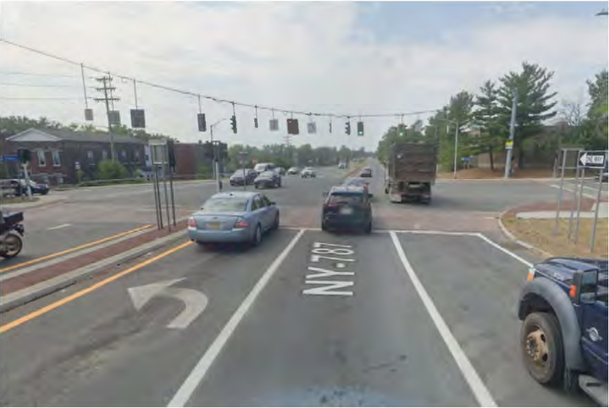
Exhibit 49: Intersection of NY State Routes 787 and 478 in Cohoes, NY is a raised intersection. (Source: Google Maps Streetview)
