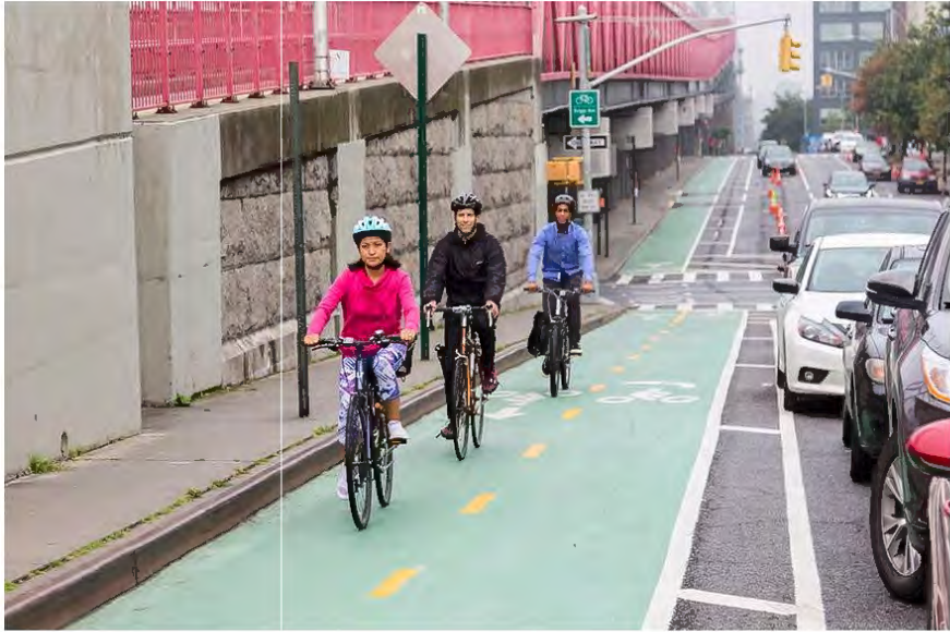
Exhibit 50: A two-way separated bike lane (also known as “cycletrack”) in New York City (Source: NYCDOT)
