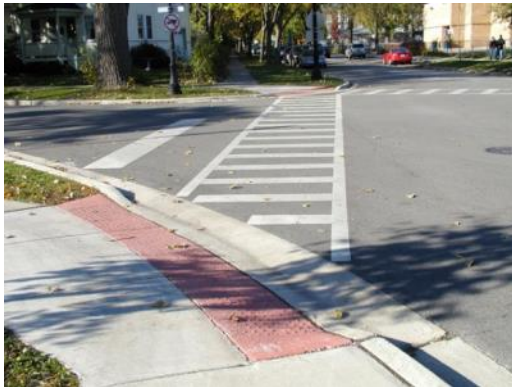
Figure 21. ADA Compliant Ramp
