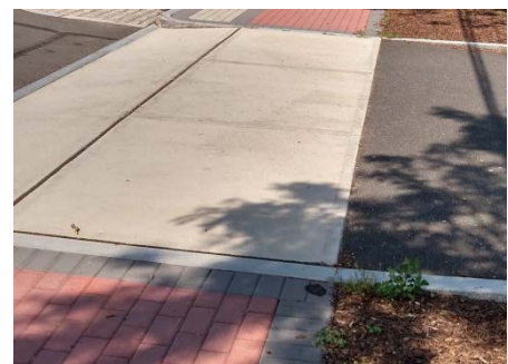
Figure 13. Driveway with Crosswalk Giving Pedestrians the Right of Way
