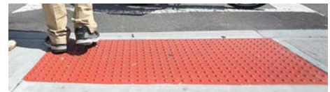
Figure 27. Tactile Warning Strip
