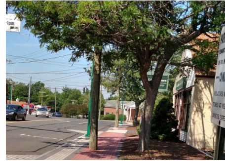
Figure 12. Utility Pole in the Middle of the Sidewalk
