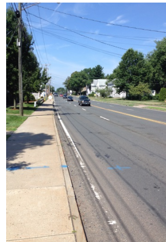
Figure 18. Sidewalk on the South Side of Route 175
