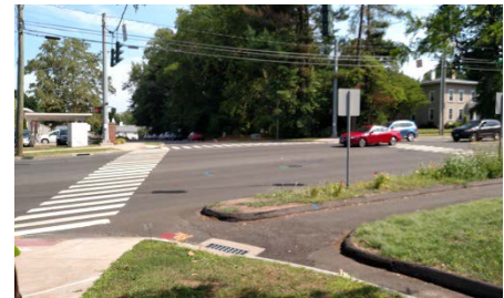
Figure 6. Traffic Signal at the Senior Center
