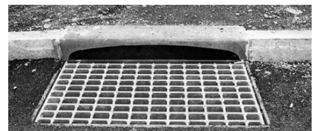
Figure 28. Example of Bicycle Friendly Catch Basin
