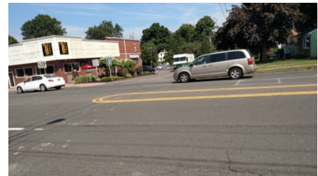
Figure 21. Painted Median Extends into Intersection
