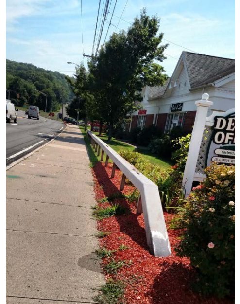
Figure 17. Lack of Buffer/Snow Shelf on the South Side of Route 175
