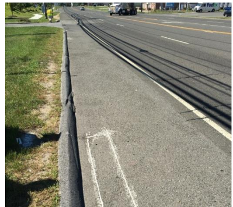
Figure 10. Section of Wider Shoulders on Route 7
