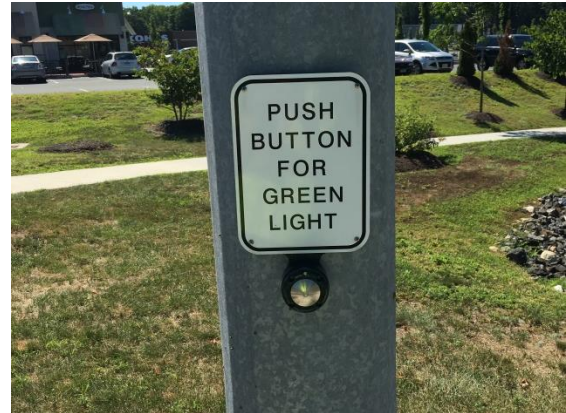
Figure 6. Pedestrian Pushbutton at Dodd Road
