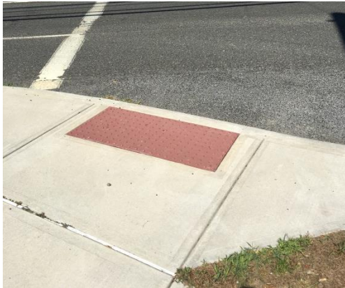
Figure 5. Ramp and Detectable Warning Strips
