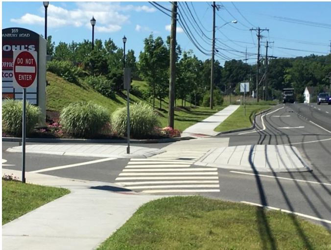
Figure 7. Crosswalk at Kohl's Plaza
