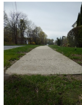
Figure 14: Sidewalk south of Bear Mountain Road
