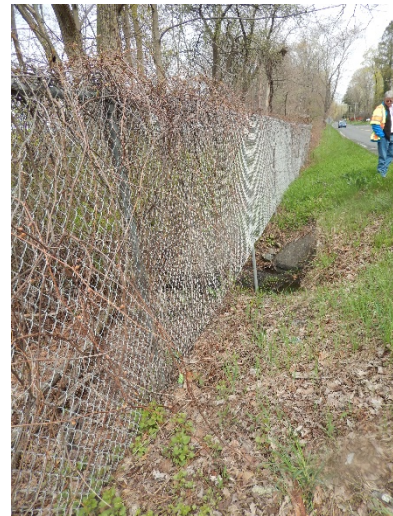
Figure 15: Culverts along Route 37
