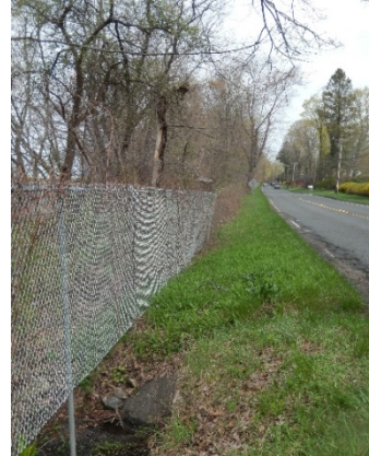
Figure 12: west side of Route 37 north at Reservoir View Drive
