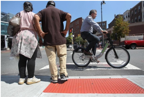
Figure 9: ADA Compliant Ramp
