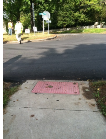
Figure 7. Sidewalk Ramp at East St. Intersection
