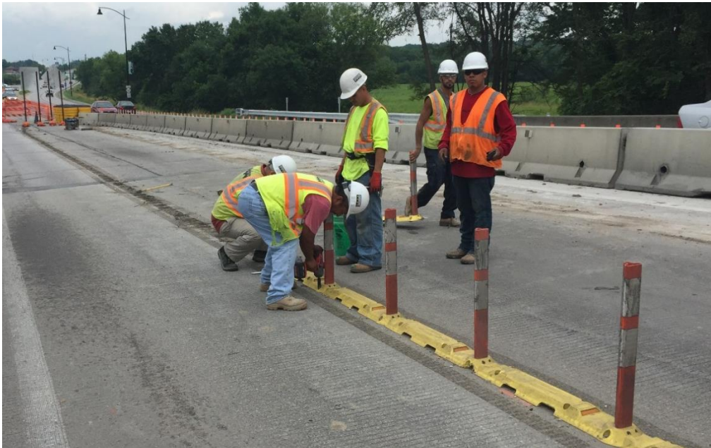
Figure 1. Temporary bollards being detached by workers
