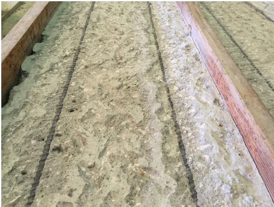
Figure 44. Positive bending flexural test specimen after roughening of substrate concrete (Case 1)
