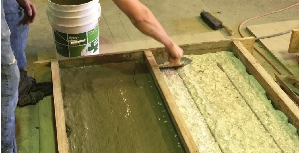
Figure 45. Application of grout to positive bending flexural test specimen (Case 1)
