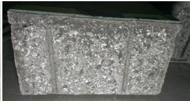
c) Bond interface (overlay concrete)
