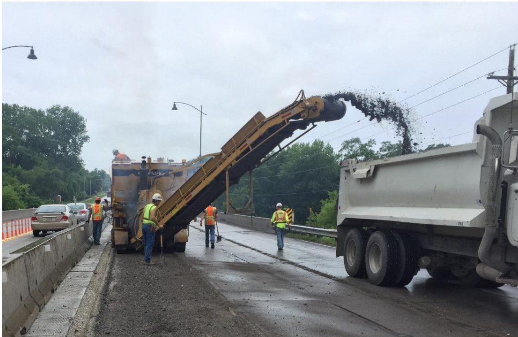
Figure 2. Milling machine removal of top layer of the deck
