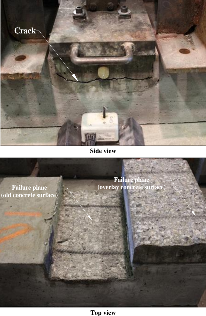
Figure 16. Case 1 pull-off test specimen failure at concrete bond interface
