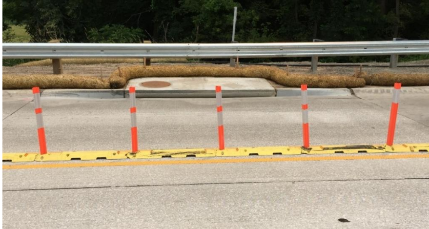
Figure 7. Manhole discovered near the approach to the westbound lane
