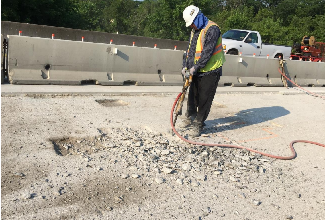
Figure 4. Removal of unsound concrete using jackhammer
