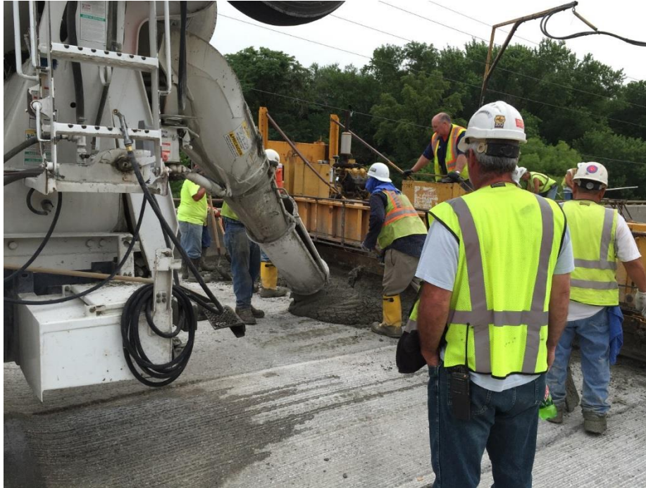
Figure 6. Ready-mixed concrete being placed on the deck
