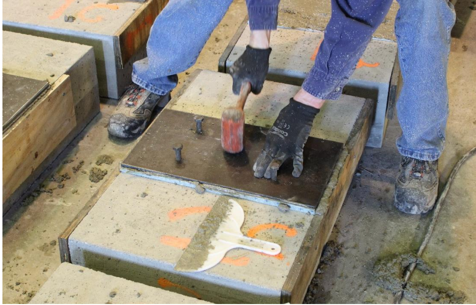
Figure 14. Tapping the steel plate to embed the shear studs on a pull-off test specimen
