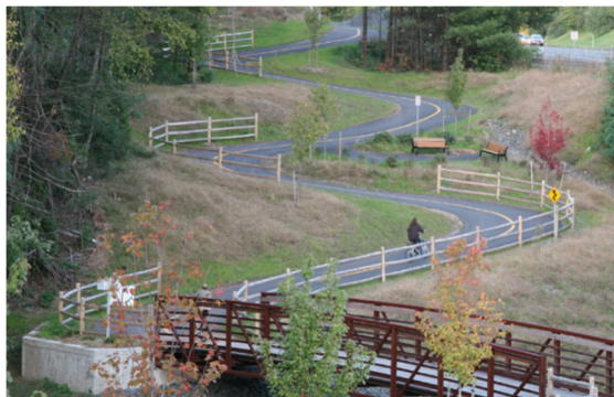
Figure 7: Shared Use Path , Charter Oak Greenway, Manchester, CT - Image Credit: CTDOT. A shared use path is a facility that is shared by bicyclists and pedestrians. These facilities are recreational in nature and often travel through open space areas and along natural features such as riverfronts. While similar in design and function to a side path, shared use paths, are not typically located adjacent to a roadway.
