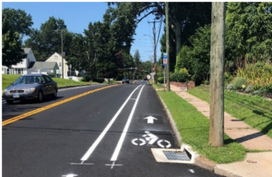
Figure 3: Typical Buffered Bicycle Lane , West Hartford, CT - Image Credit: FHI Studio. Buffered bicycle lanes are conventional striped bike lanes with a painted or textured pavement buffer space that is used to separate the bike lane from the adjacent motor vehicle lane and/or parking lane.
