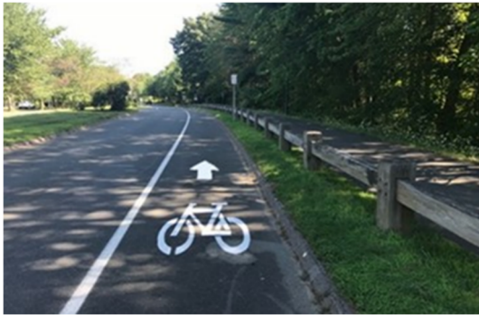
Figure 2: Typical Bicycle Lane , Simsbury, CT - Image Credit: FHI Studio: Bike lanes designate an exclusive space on the roadway for bicycle travel, which is signified by pavement markings and signage. Bike lanes are typically located between a motor vehicle travel lane and the curb, road edge, or parking lane.
