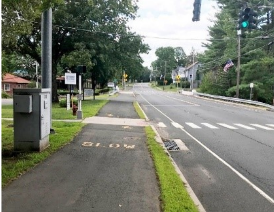
Figure 5: Side Path , Farmington Canal Trail, Simsbury, CT- Image Credit: FHI Studio. Side Paths provide a separated facility for the shared use of bicyclists and pedestrians. Like sidewalks, these facilities are physically separated from motor vehicles by a curb, open space, or barrier. These facilities are adjacent to the roadway and are typically located within the right-of-way.
