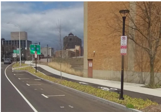
Figure 6: Separated Bicycle Lane - 1-way at Sidewalk Level , New Haven, CT – Image Credit CTDOT Photolog. Separated Bike Lanes (also known as cycle tracks or protected bike lanes) are bicycle lanes that are physically separated from motor vehicle traffic. Separated bike lanes can be designed for one-way or two-way travel and can be at street level, at sidewalk level, or at an intermediate level between the two.
