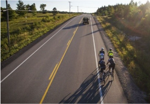
Figure 1: Paved Outside Shoulder , -Image Credit: Clay Dolan. Paved outside Shoulders designate a shared space on the roadway for bicycle travel. Paved Outside Shoulders are typically located between a motor vehicle travel lane and the curb or road edge.
