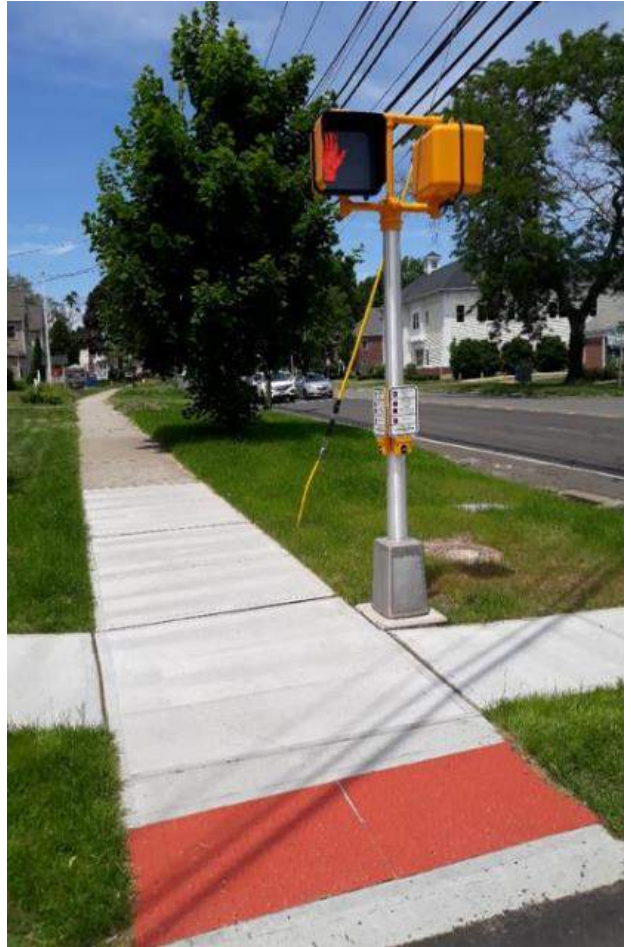
Figure 27 – APS Signal and Curb Ramp
