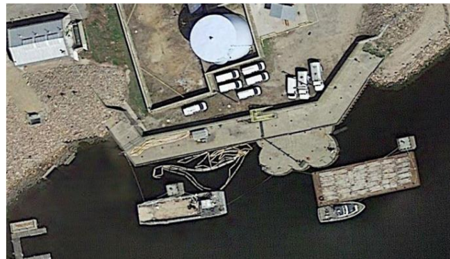
Shaw's Cove Pump Station Steel Pile Wall Reconstruction, New London
