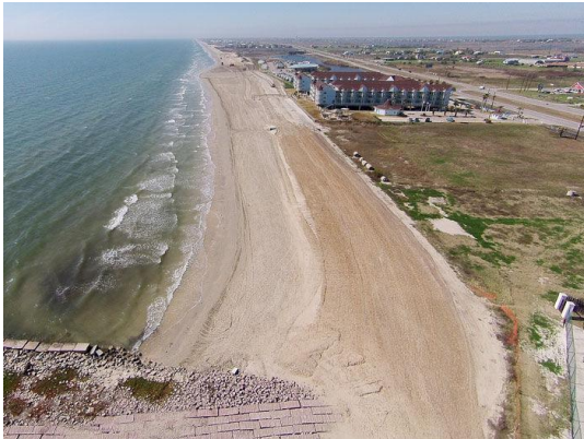
Beach Street Reconstruction West Haven
