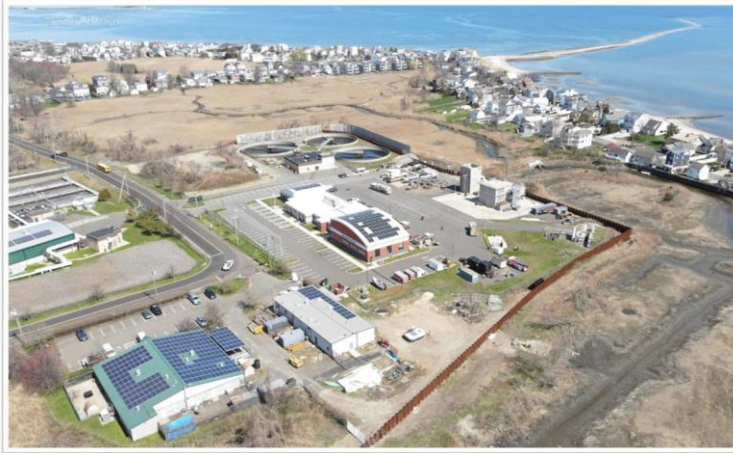
Wastewater Treatment Plant Resiliency Fairfield
