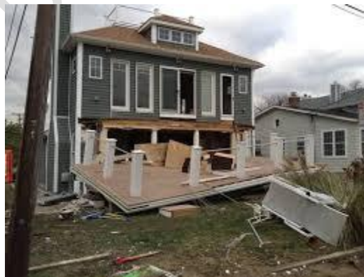
Norwalk Damage (USA Today; Oct 31, 2012)
