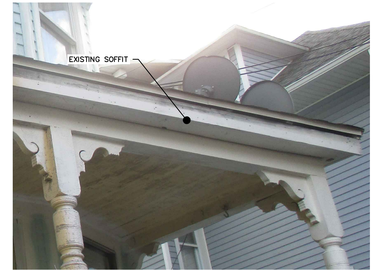
PHOTO 2 (EXISTING CORBEL AND PINE BOX TRIM TRANSOM)
