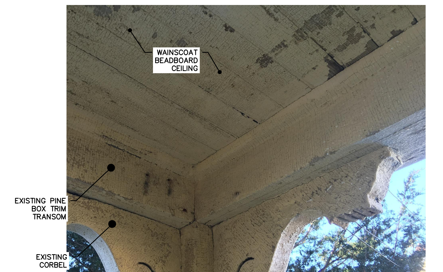
PHOTO 4 (EXISTING WAINSCOT CEILING, QUARTER ROUND TRIM, PINEBOX TRIM, AND PARTIAL CORBEL)
