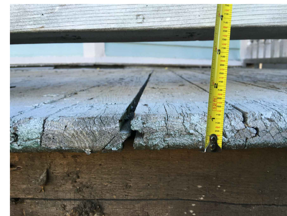
PHOTO 3 (EXISTING 5/4 BY 4 SQUARE EDGE TONGUE AND GROOVE BOARD DECKING)
