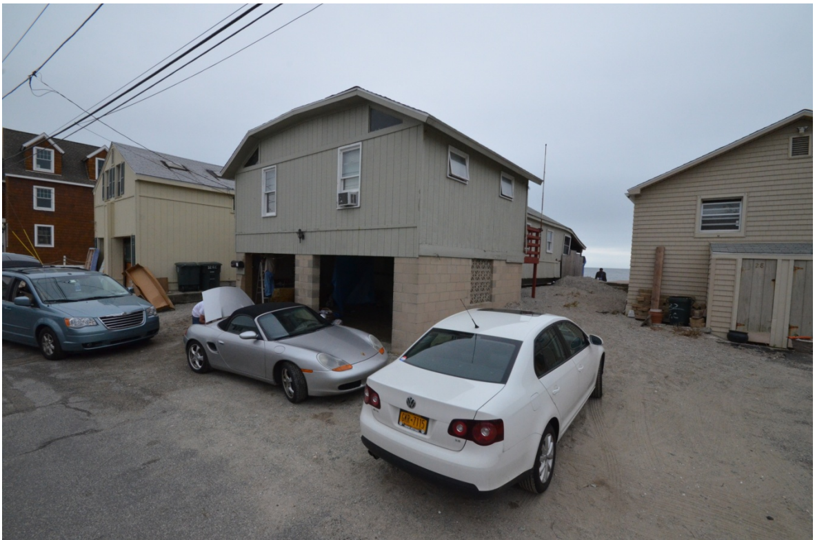
Figure 10 view of site from street
