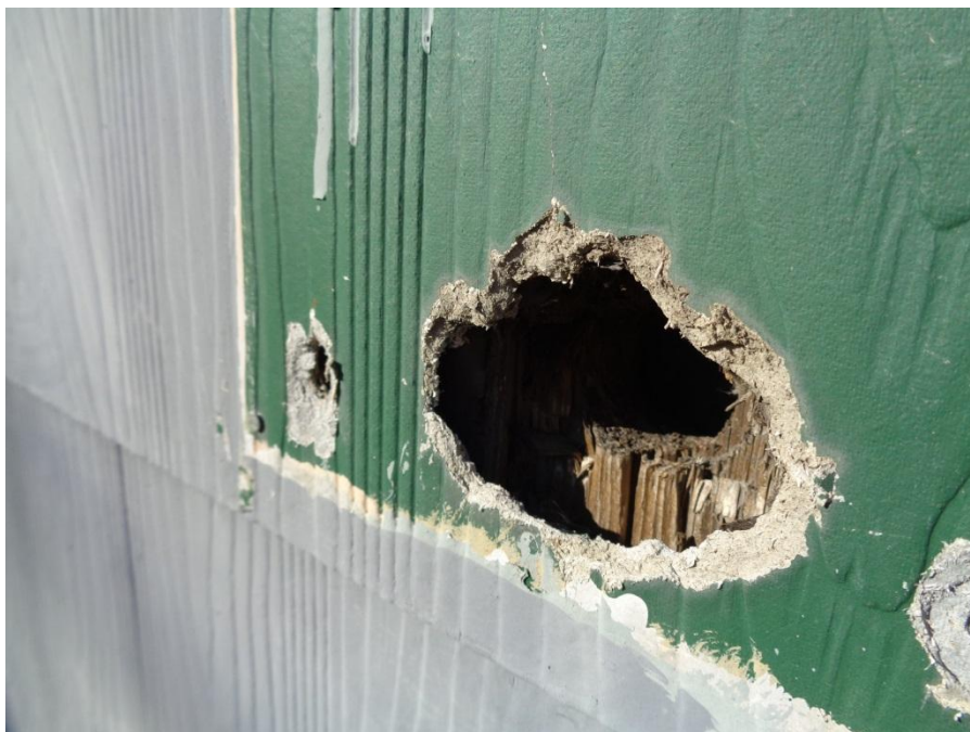
Opening in ACM Exterior Gray Cementitious Panel Siding
