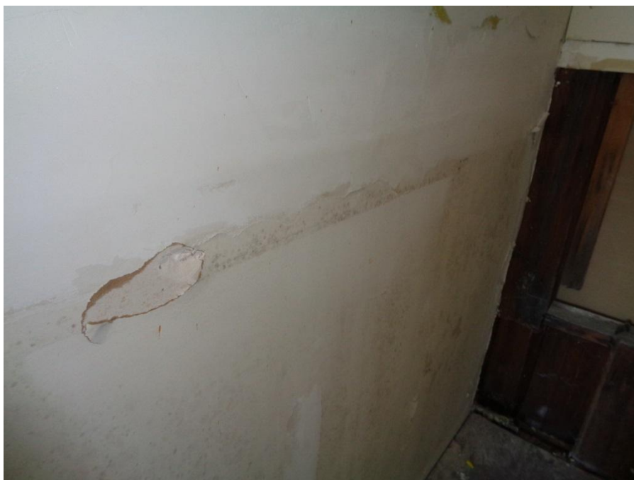
Mold Growth on Sheetrock Wall, Furnace Room
