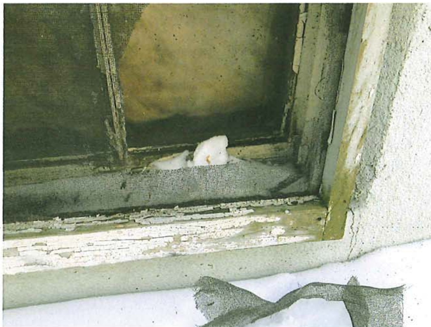
Typical North Basement Window
