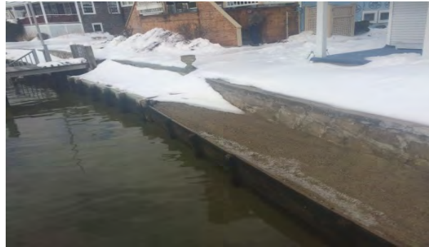
Photo 5: Seawall on site and adjacent properties; looking W.
