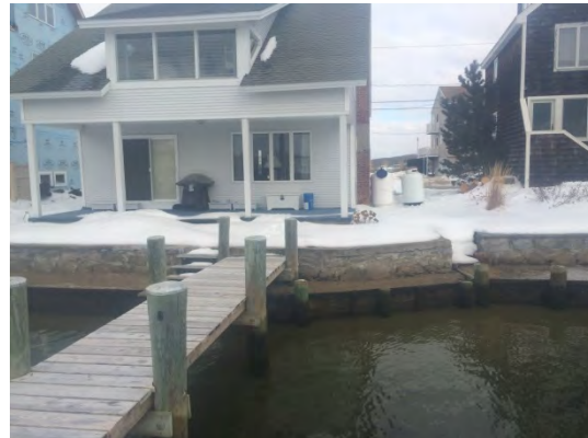
Photo 6: Eastern side of property; looking N. Note seawall on eastern side of the dock.
