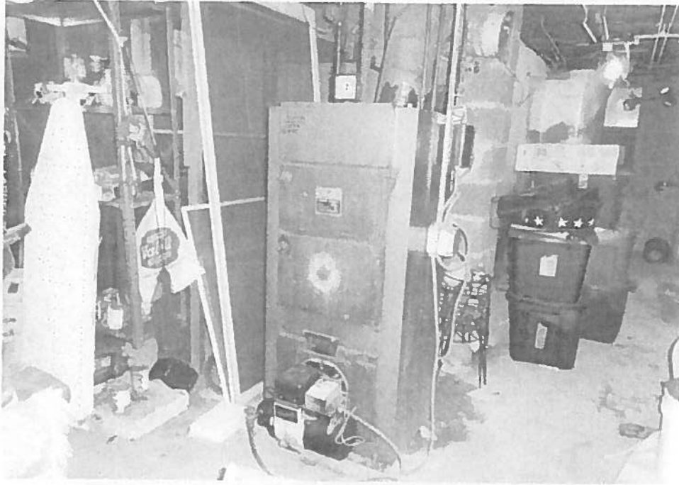
Inaccessible Furnace: Interior Materials Presumed to be ACM
