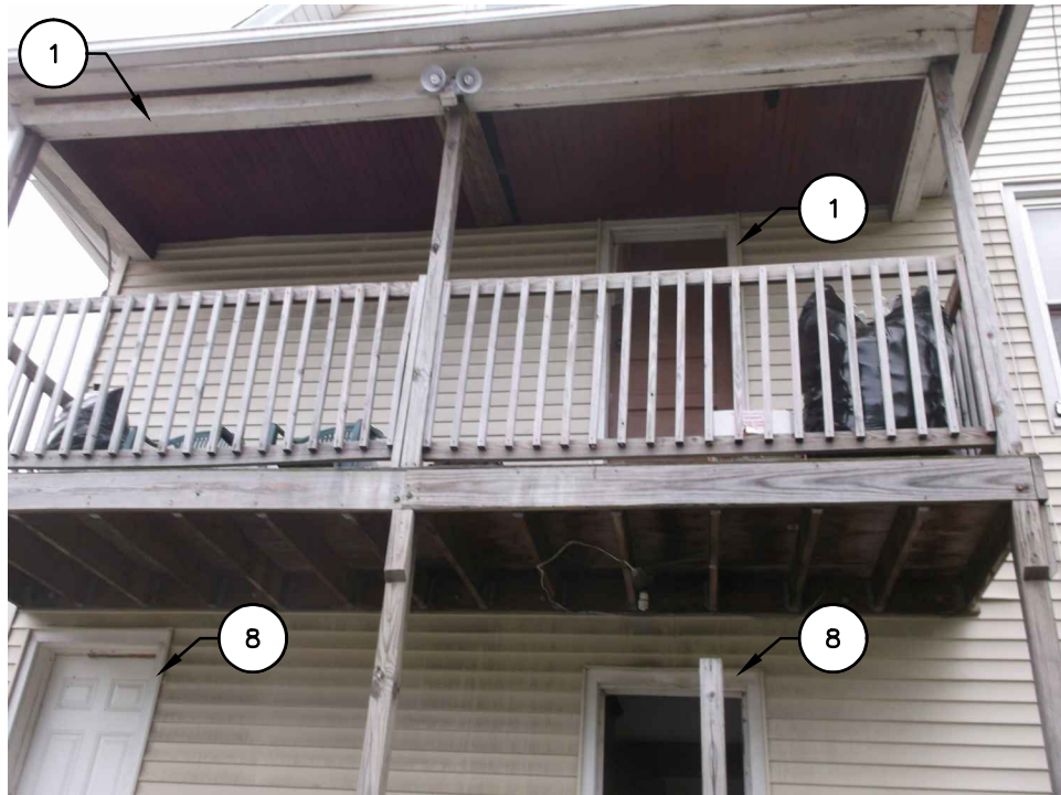
PHOTO 1 REAR PORCH – FIRST AND SECOND FLOOR (N.T.S.)
